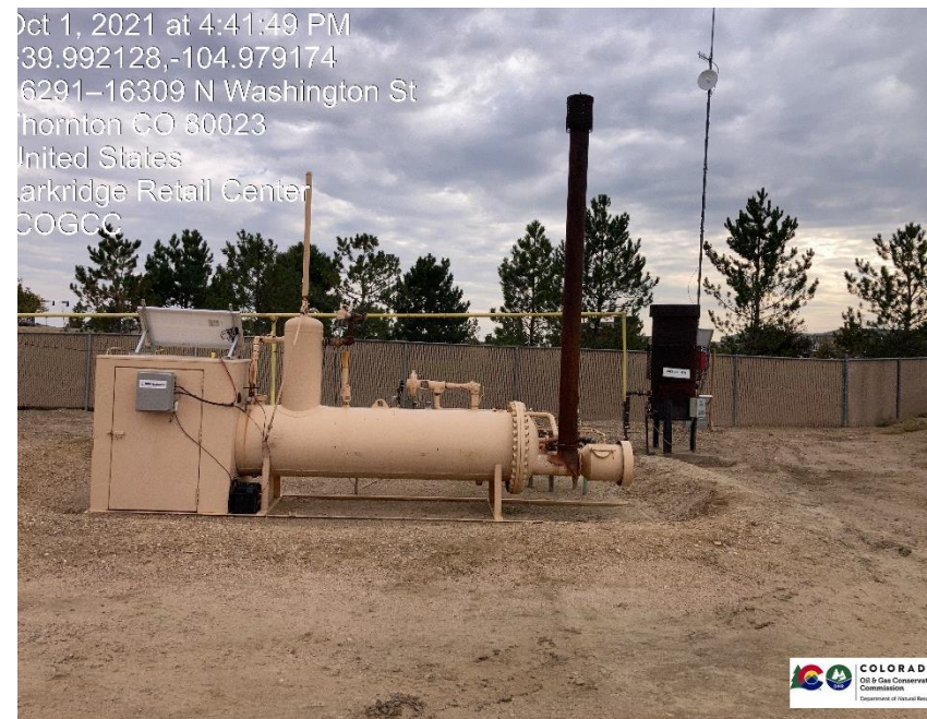
Pic 4 separator, ECD. Automation equipment.
