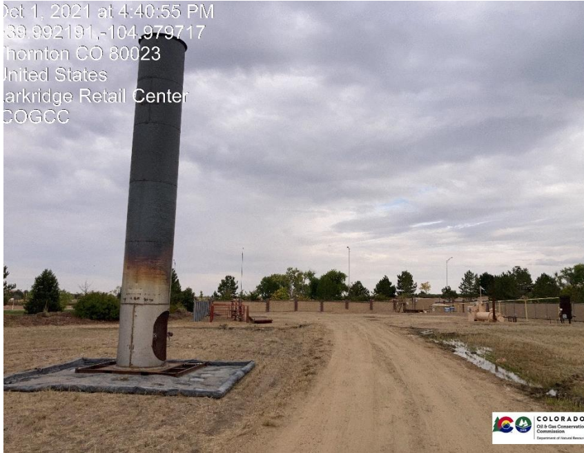
Pic 1 ECD not connected to well.
