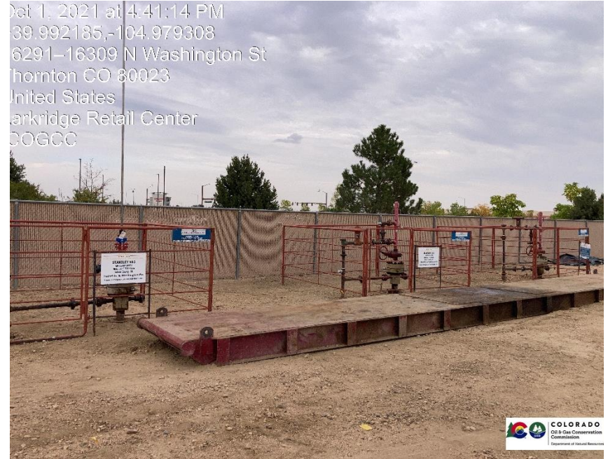
Pic 2 basebeam in front of well. Rods have been installed on first well, no rig on location.
