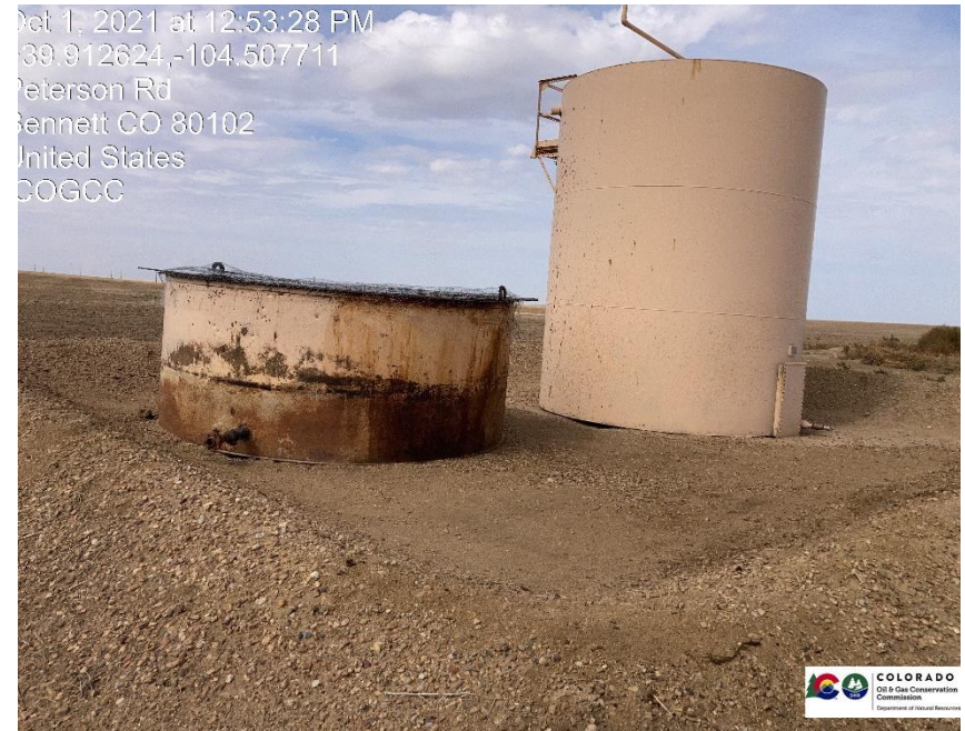
Pic 2 open top tank does not have labels
