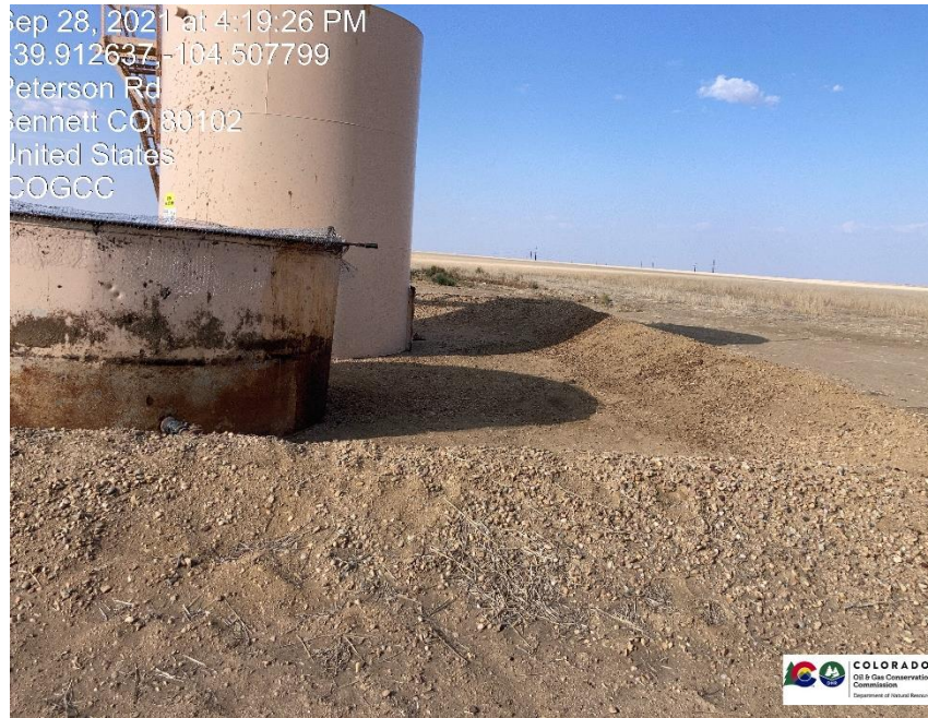
Pic 1 tanks, open top tank does not have labels
