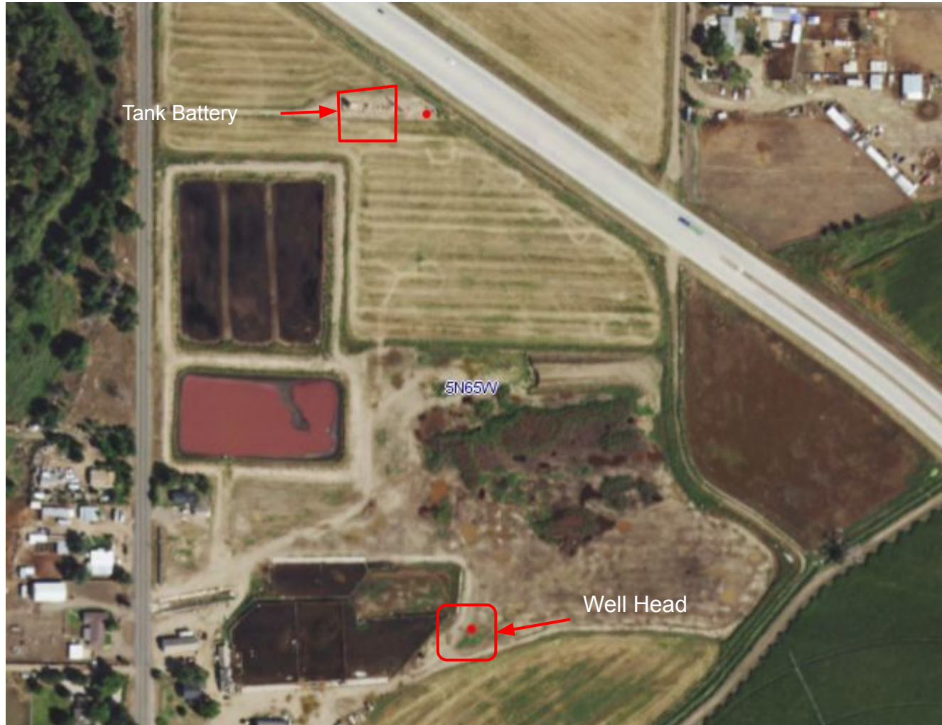
Photo 1. 2019 aerial imagery shows the well head and tank battery (north is up). Note: no well head access road (well was accessed via farm road). The tank battery is still in operation and is associated with API#123-11892.
