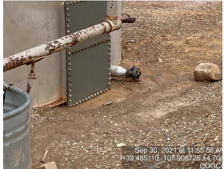
Missing bull plug/caps on load out lines
