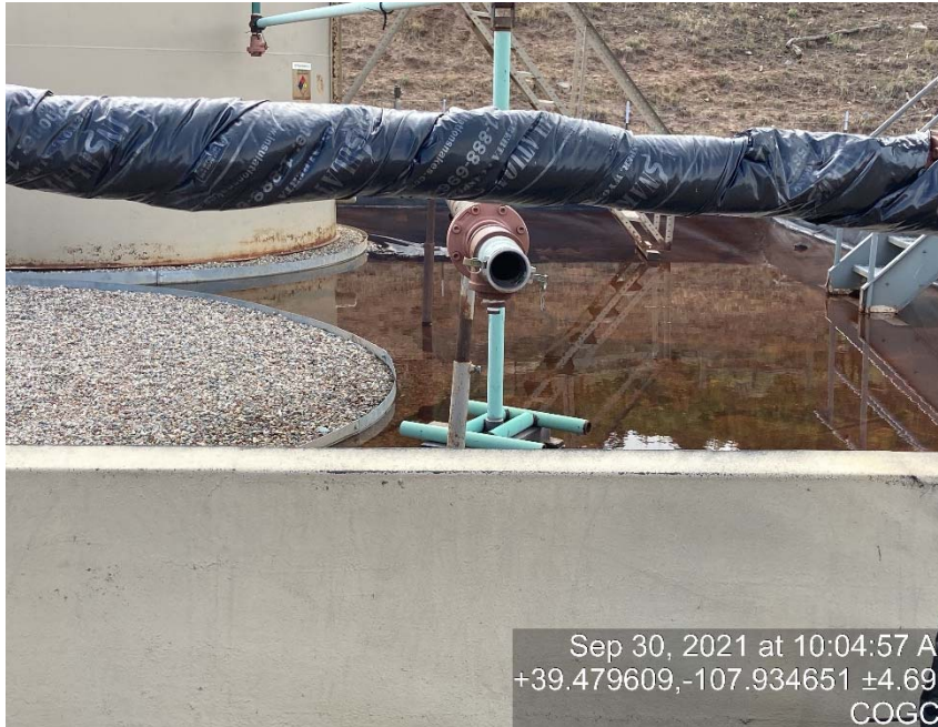
Missing bull plug/caps on load out lines
