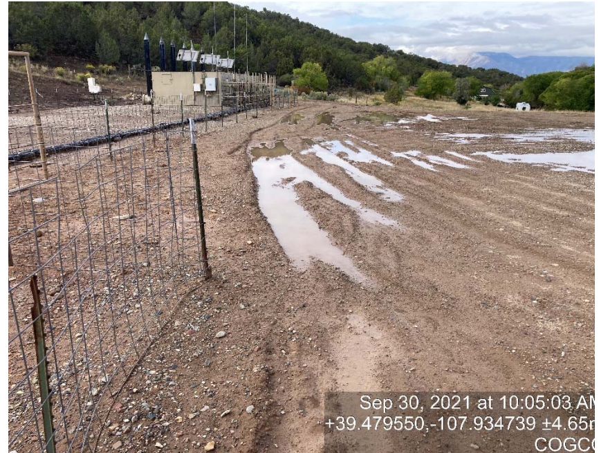
Lack of stabilization/compaction
