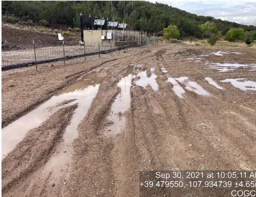
Lack of stabilization/compaction
