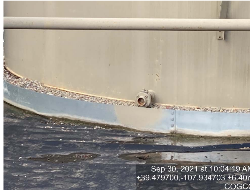
Missing bull plug/caps on load out lines
