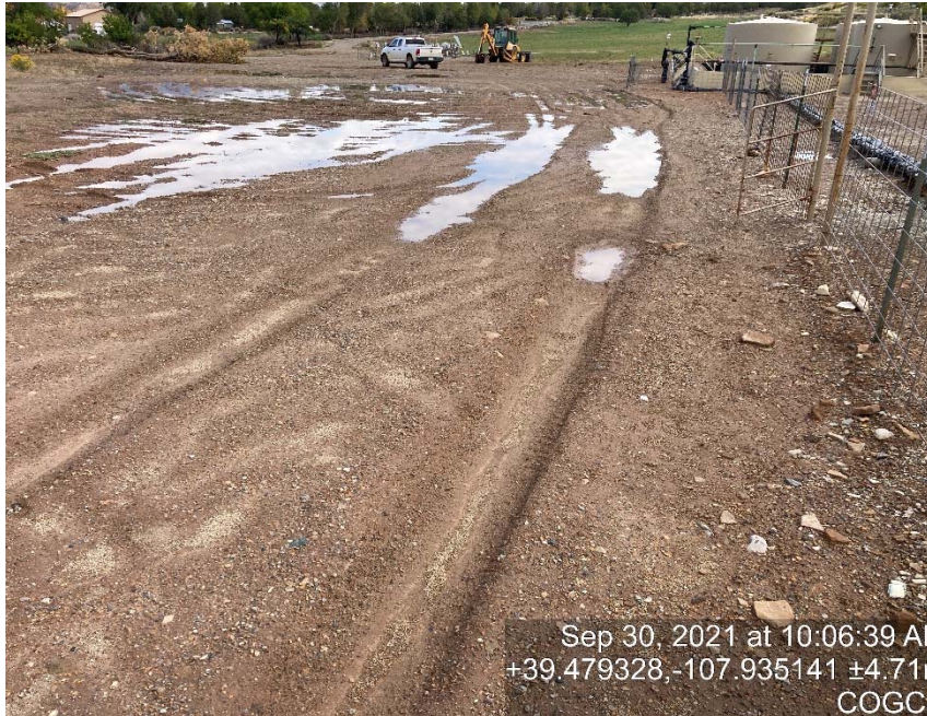
Lack of stabilization/compaction
