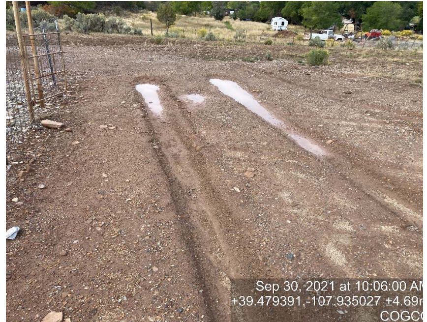
Lack of stabilization/compaction
