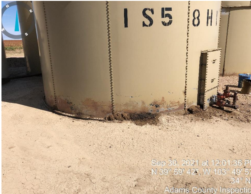
Photo # 11 South West side of crude tank, stained soil from leaking tank.
