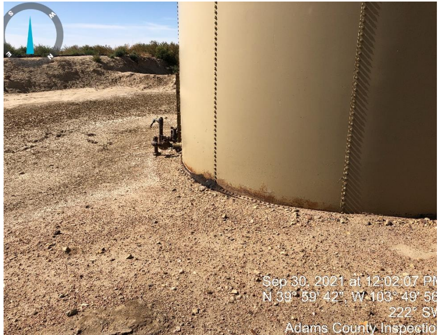
Photo #14 East side of East crude tank, stained soil from leaking tank.
