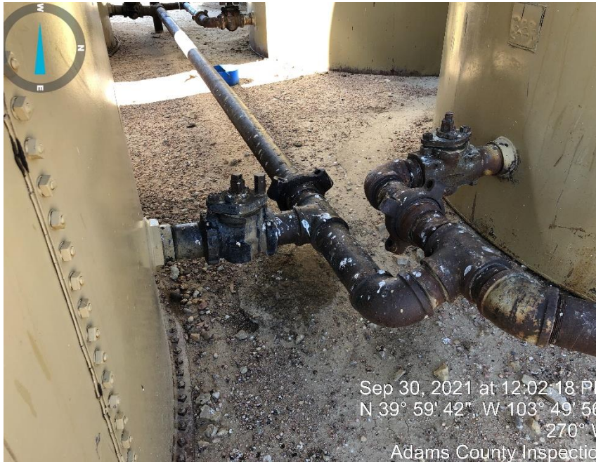
Photo #15 stained soil under valves in-between crude tanks
