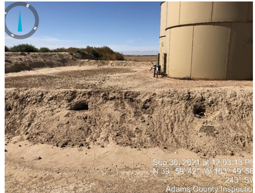
Photo #18 East side of unmaintained berm around tanks.
