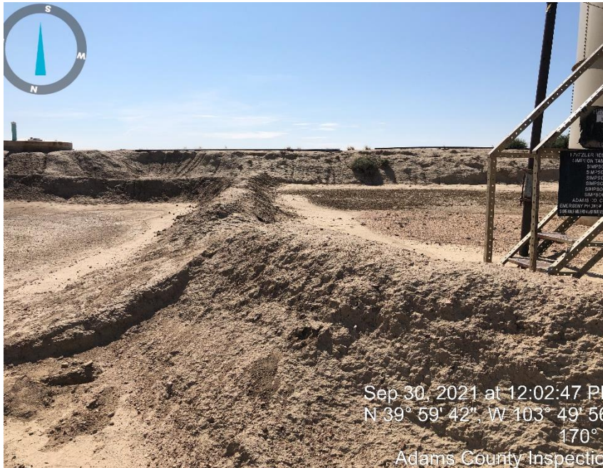
Photo #19 West side of unmaintained berm around tanks
