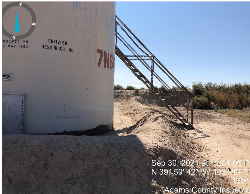
Photo #17 West side of unmaintained berm around tanks.
