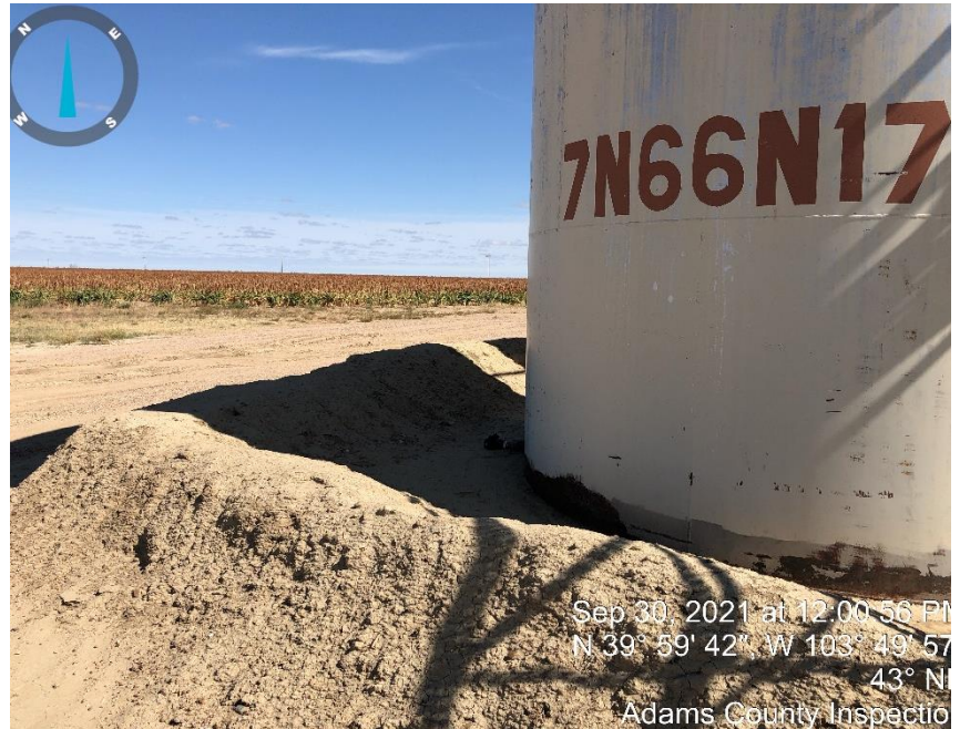
Photo #16 West side of unmaintained berm around tanks.
