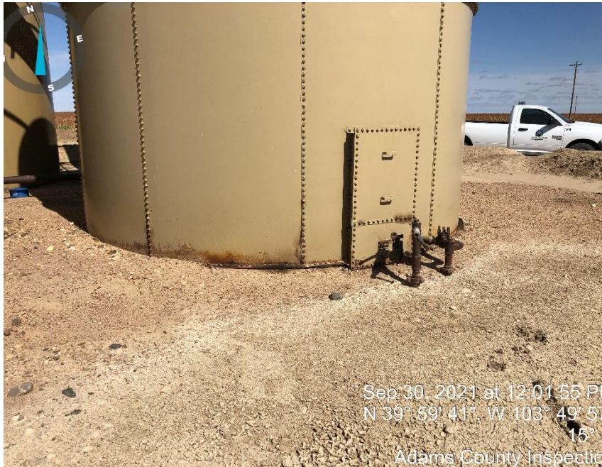
Photo #13 South West side of East crude tank, stained soil from leaking tank.
