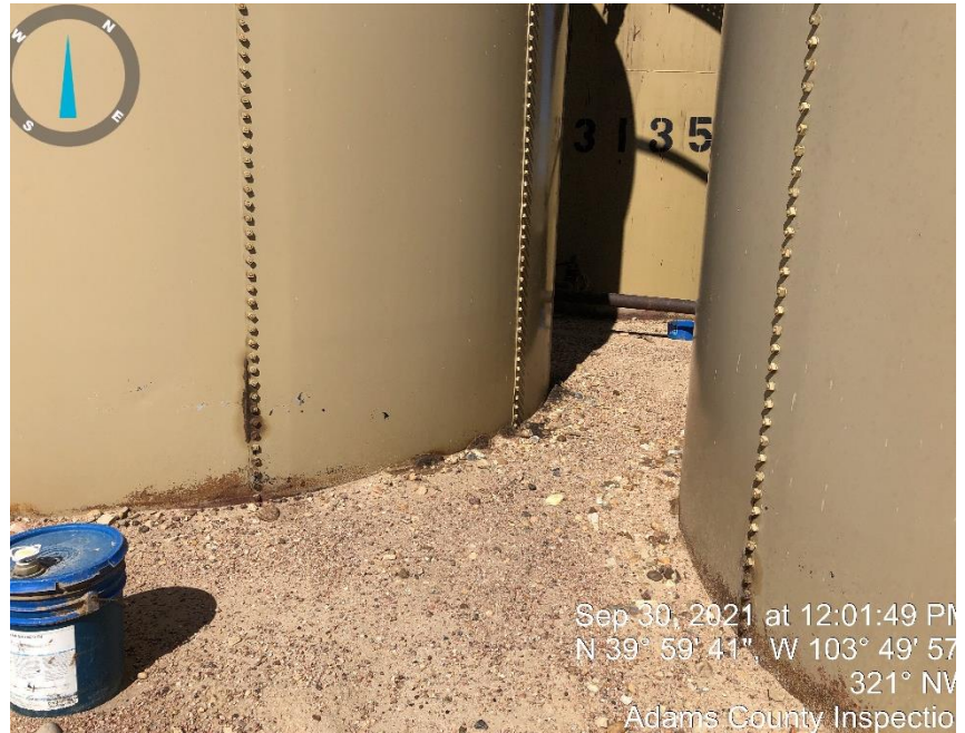
Photo #12 South side of crude tank, stained soil from leaking tank.
