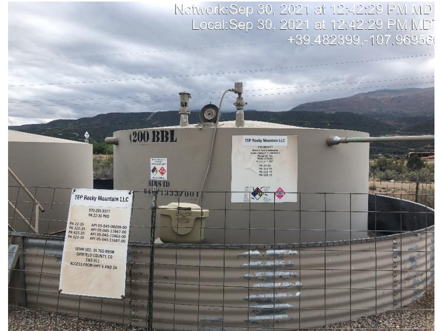
Photo #4983 Gauge hatch open.
