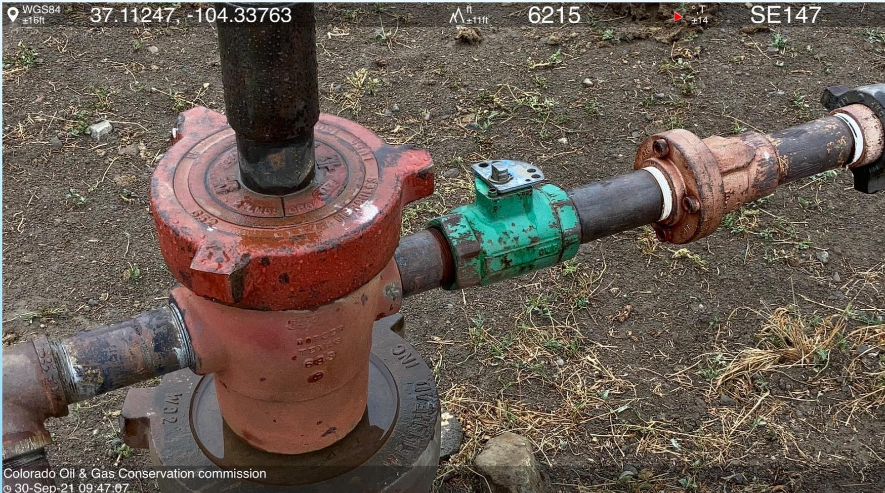
PHOTO 4: CSG/TBG ANNULUS IS SI. VALVE IS NOT LOTO.
