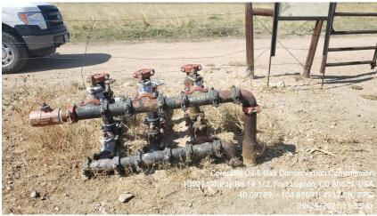
Photo 7 Stained soil by crude oil tank load out line.
