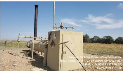
Photo 11 Stained soil by the Gas Meter Run
