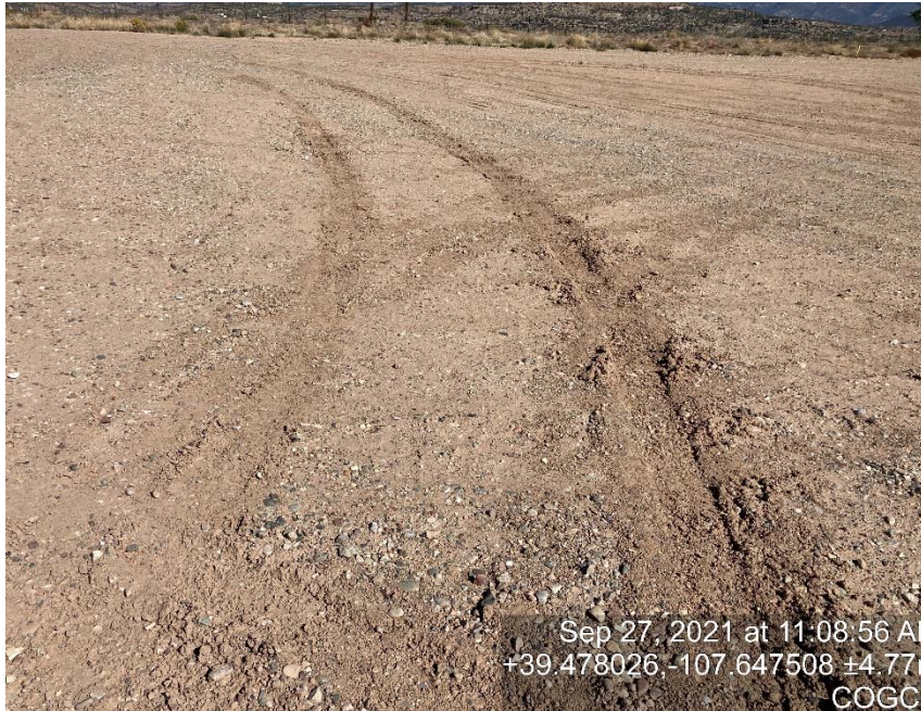
Lack of stabilization/compaction
