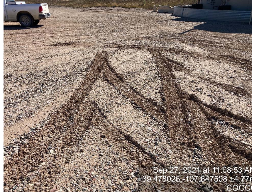
Lack of stabilization/compaction
