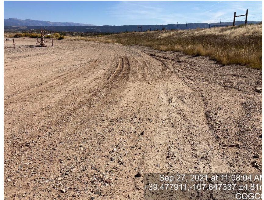
Lack of stabilization/compaction
