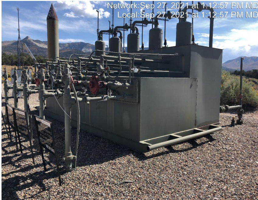
Photo #4964 Glycol storage tank missing required information.
