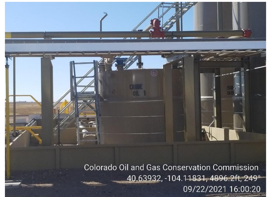
Photo 8 – Capacity Label missing
