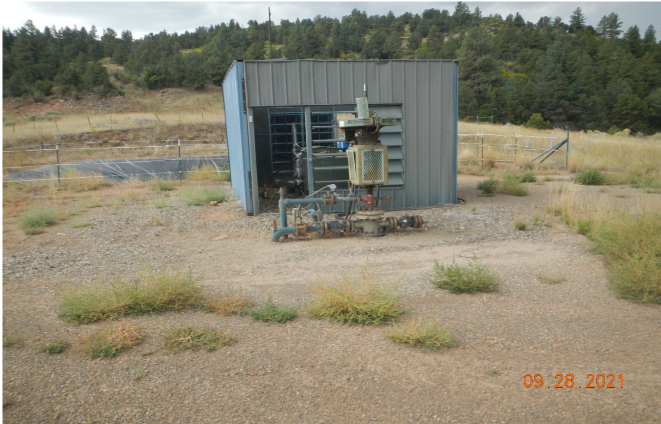
Photo 2. Facing toward the well and pit which is lined and fenced.
