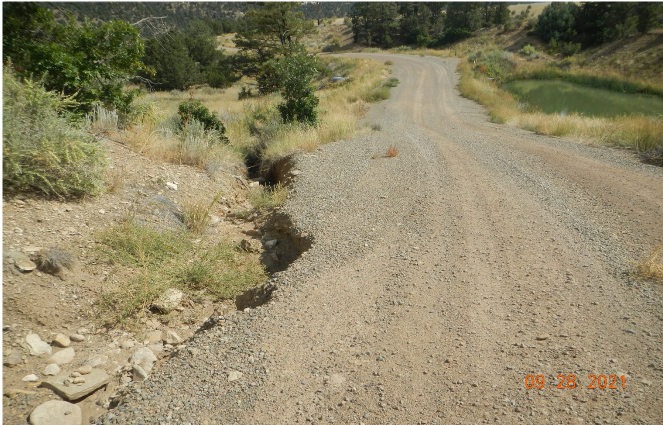
Photo 2. The erosion continues off the side of the road shown from previous photo. This area needs to be stabilized.
