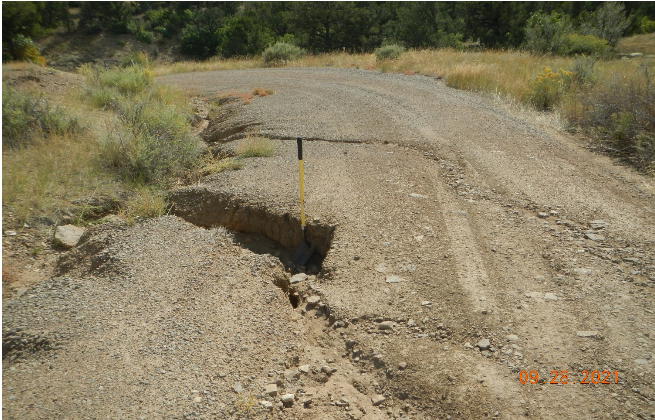
Photo 1. There is erosion along the access road near the location. Areas of erosion need to be repaired and stabilized. Previous corrective action was not performed.
