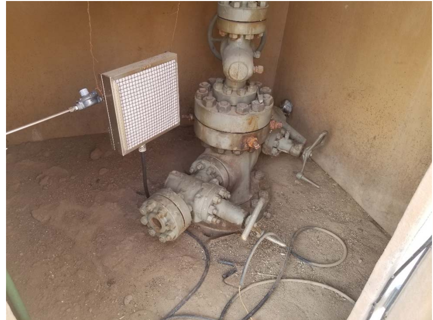
Photo 3. No bradenhead access apparent.
