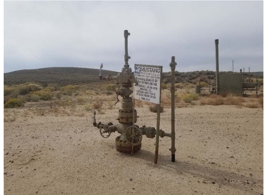
Photo 2. No bradenhead access apparent. Previous operator on location signs.
