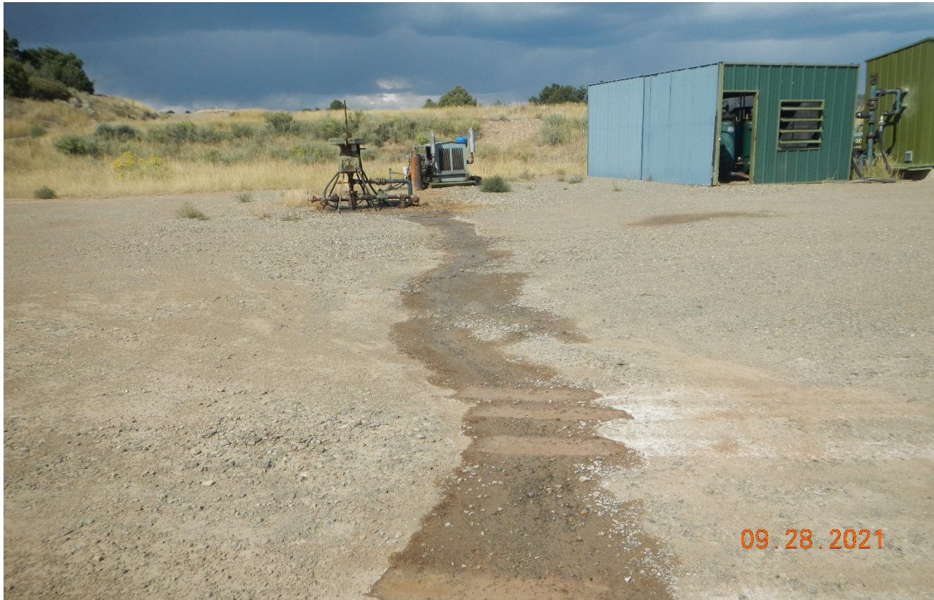
Photo 2. There is a dripping water leak at the wellhead causing water to spill across the location.
