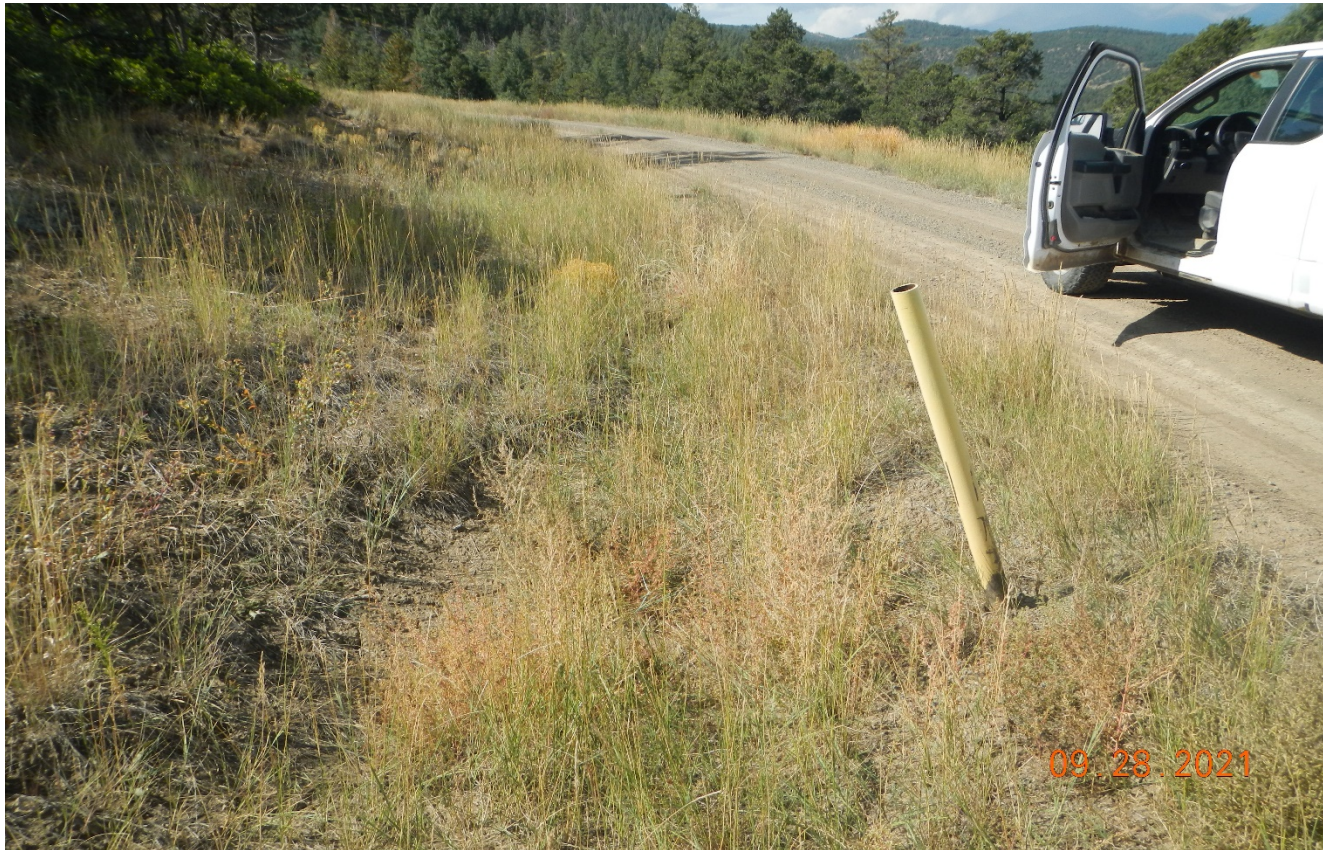
Photo 2. Facing west along access road. The culvert is filled in with sediment and stormwater from the road is not being directed toward the culvert from the road.
