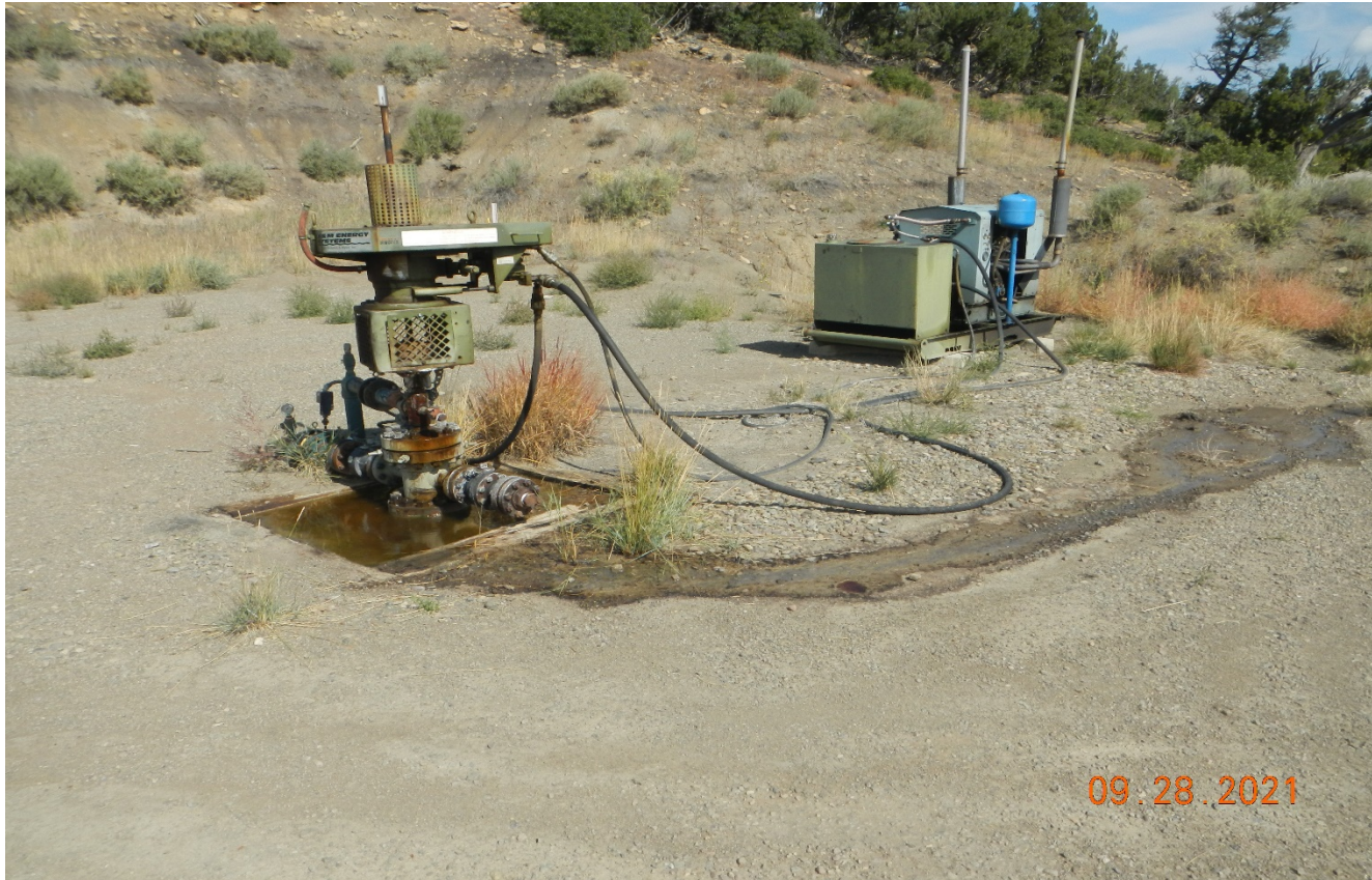
Photo 6. There is a dripping water leak at the wellhead which has not been repaired.
