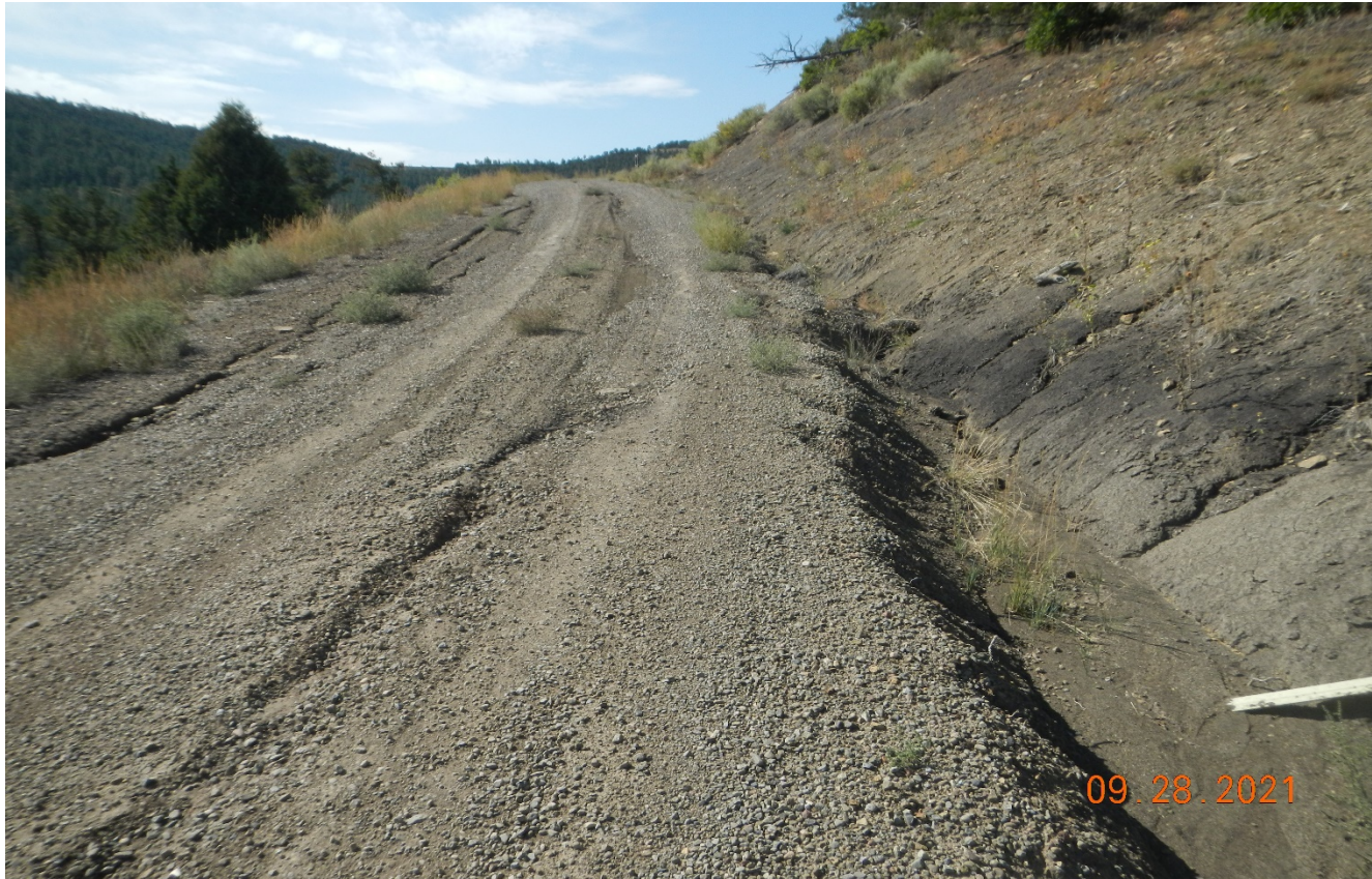
Photo 4. There is erosion along the side of the road which needs BMP's to prevent further erosion.
