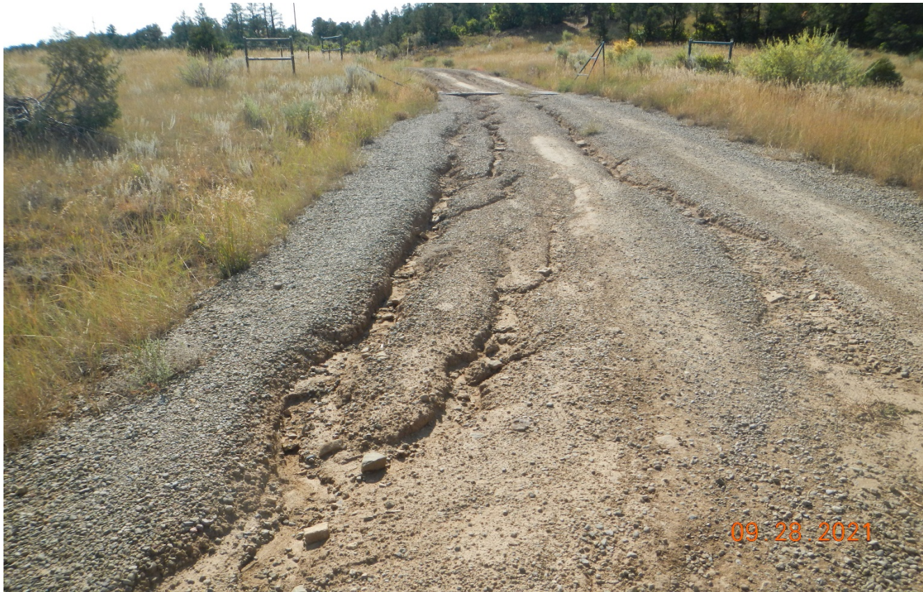
Photo 1. Facing southeast along the main access road. The erosion along the road needs to be repaired. Previous corrective action was not completed.
