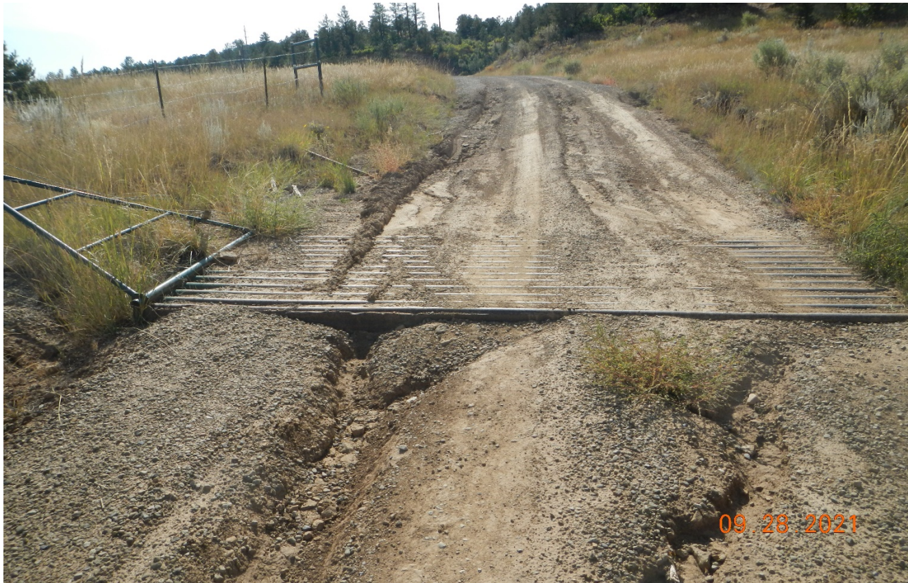
Photo 2. The cattle guard is filled in with sediment and needs to be repaired. Previous corrective action was not completed.
