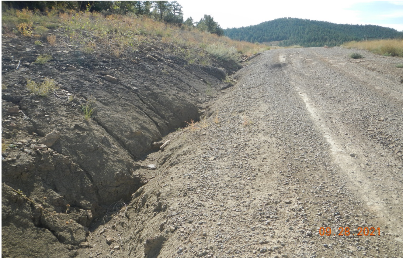
Photo 3. There is erosion along the side of the road which needs BMP's to prevent further erosion.
