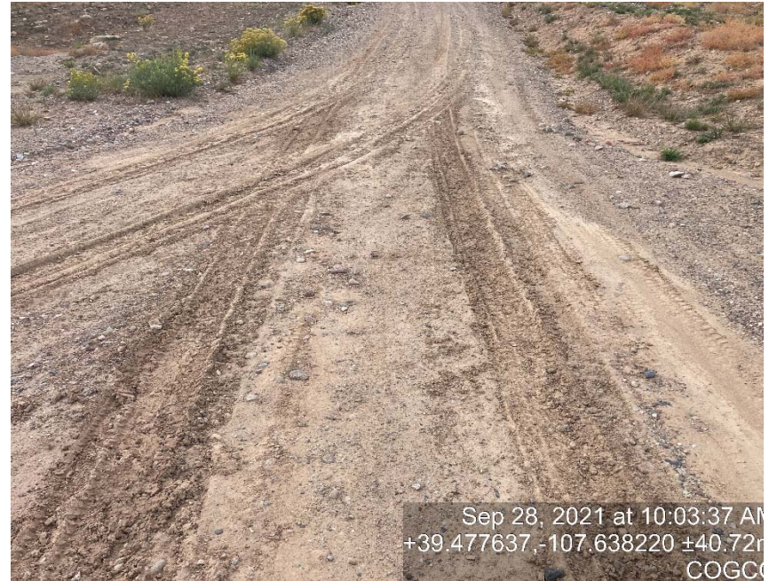
Lack of stabilization/compaction
