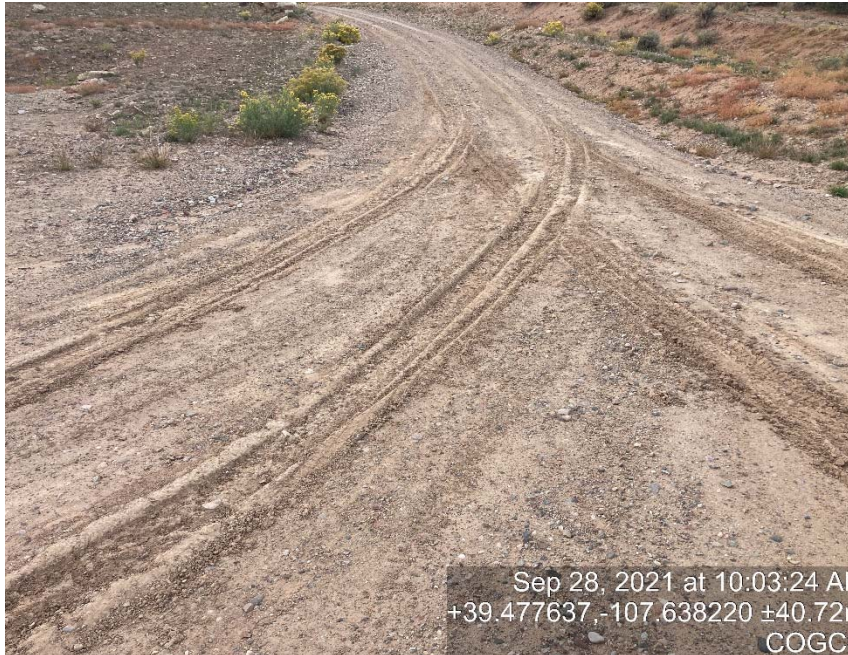
Lack of stabilization/compaction
