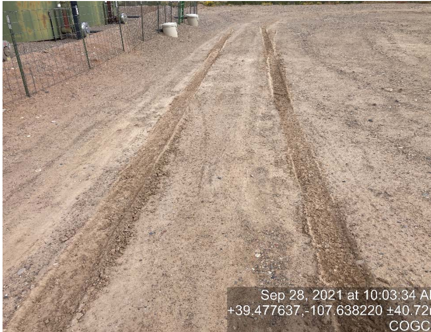
Lack of stabilization/compaction
