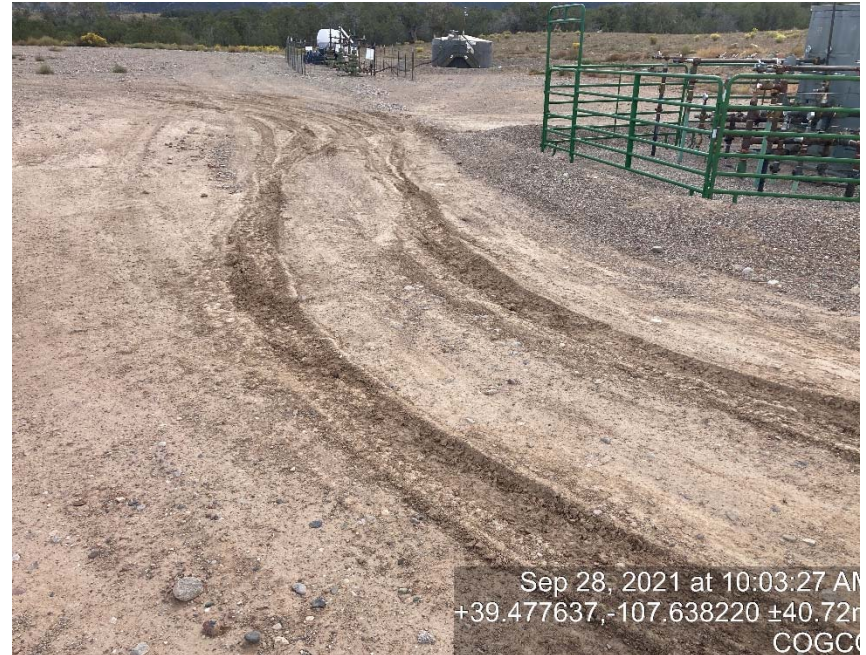
Lack of stabilization/compaction
