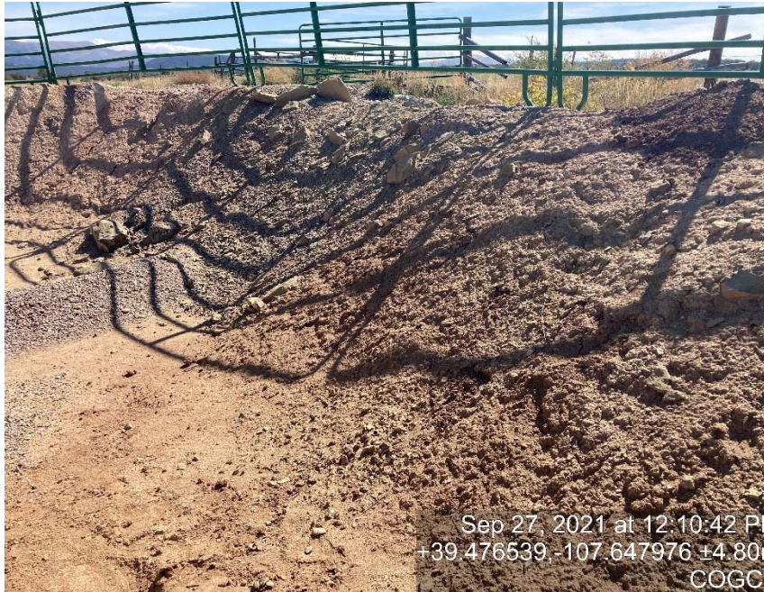
Lack of stabilization/erosion
