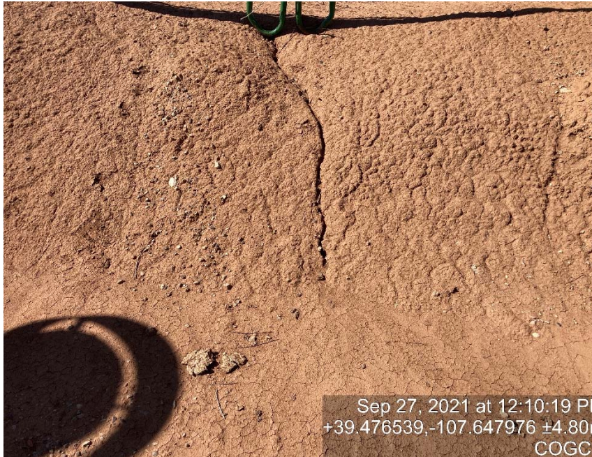
Lack of stabilization/erosion
