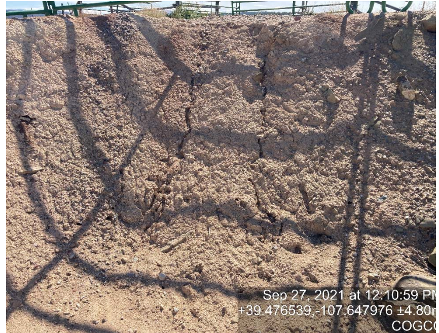
Lack of stabilization/erosion
