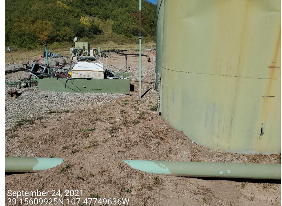
Photo 1: Photo shows adequate, impervious containment has not been installed at the tanks in accordance with good engineering practices.
