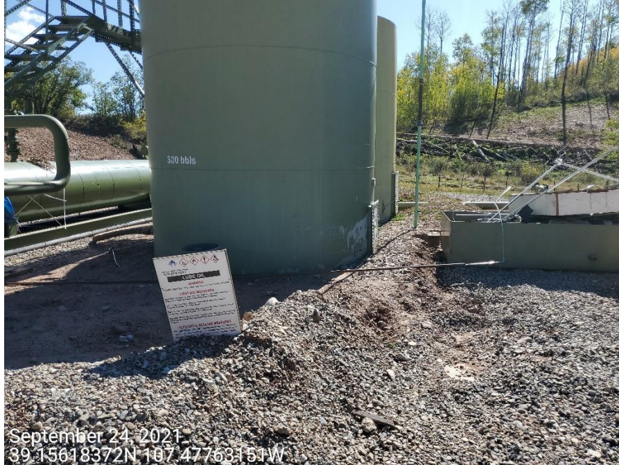
Photo 1: Photo shows adequate, impervious containment has not been installed at the tanks in accordance with good engineering practices.
