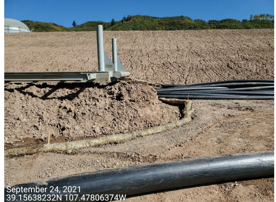
Photo 3: Photos shows control measurers at the stockpiled soil has not been installed in accordance with good engineering practices.
