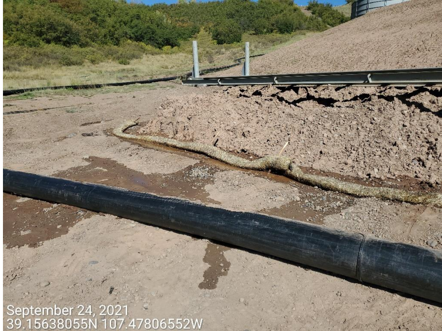
Photo 3: Photos shows control measurers at the stockpiled soil has not been installed in accordance with good engineering practices.
