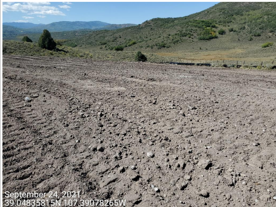
Photo 3: Photos taken from the interim areas of the Location; BMPs to stabilize soils missing or insufficient.
