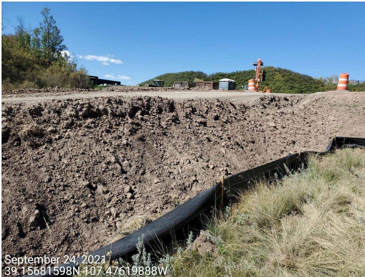
Photo 5: Photo taken from the fill slopes on the southeast end of the Location. Photo shows stormwater and erosion control measures to protect/stabilize the slopes of the Location remain missing or inadequate.
