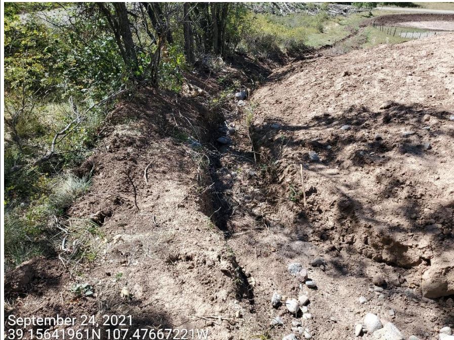
Photo 9: Photos taken from the stormwater “ditch” leaving from the Location. Photo shows section of the control that remains improperly constructed with vertical slopes with unconsolidated soils.
