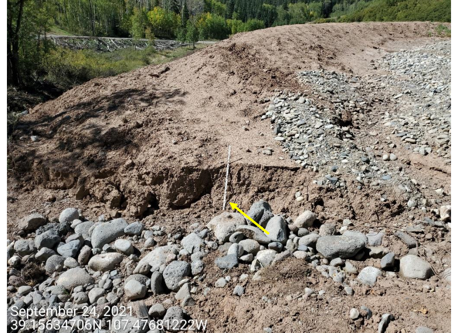
Photo 8: Photo taken from the southwest end of the pad. Photo shows that the stormwater outlets leading from the pad; erosion degradation remains evident at outlets; controls have not been installed in accordance with good engineering practices, or maintained in proper functioning condition. Two foot measuring stick for reference.
