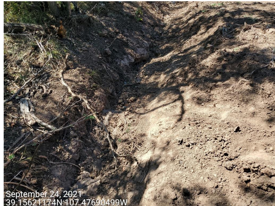
Photo 9: Photos taken from the stormwater “ditch” leaving from the Location. Photo shows section of the control that remains improperly constructed with vertical slopes with unconsolidated soils.
