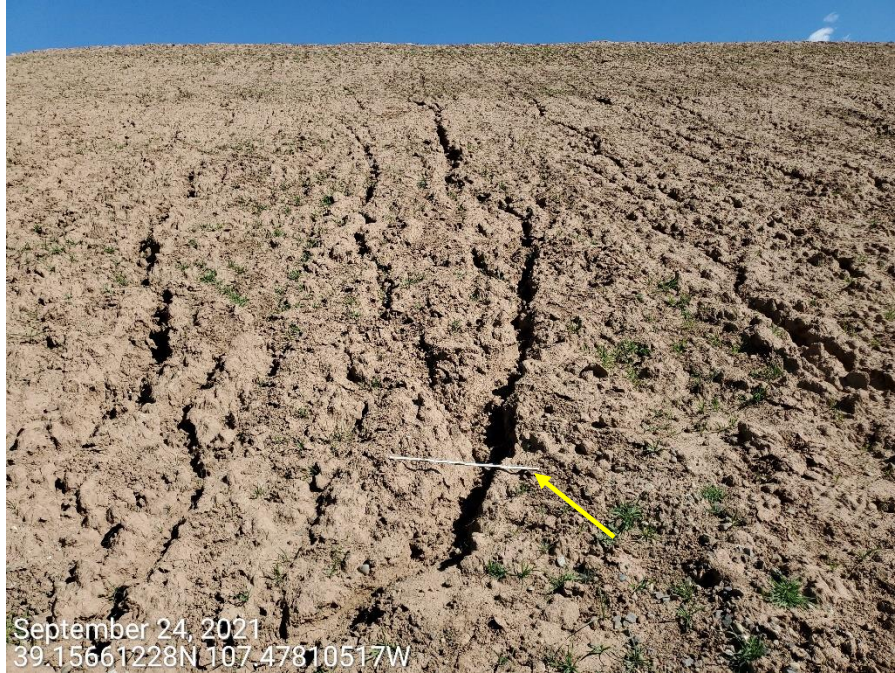
Photo 3: Photos taken from the fill slopes on the west end of the Location. Photo shows stormwater and erosion control measures to protect/stabilize the slopes of the location remain missing or inadequate. 2 foot measuring stick for reference.
