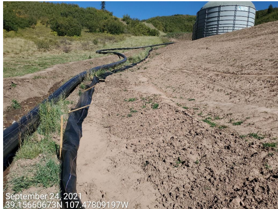
Photo 7: Photos taken from the western perimeter of the Location. Photo shows perimeter controls (silt fence) remain in improper functioning condition per good engineering practices.
