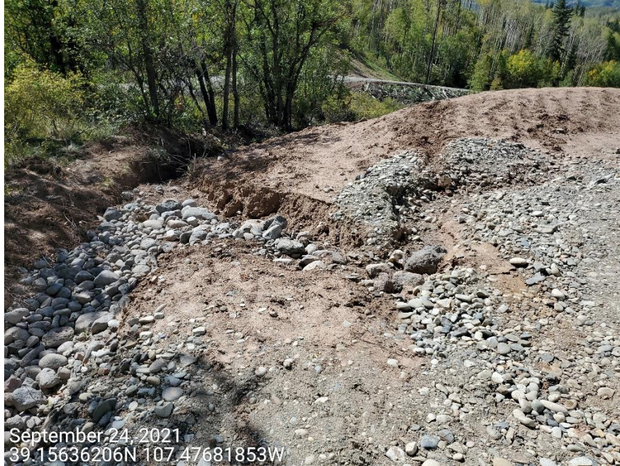
Photo 8: Photo taken from the southwest end of the pad. Photo shows that the stormwater outlets leading from the pad; erosion degradation remains evident at outlets; controls have not been installed in accordance with good engineering practices, or maintained in proper functioning condition. Two foot measuring stick for reference.
