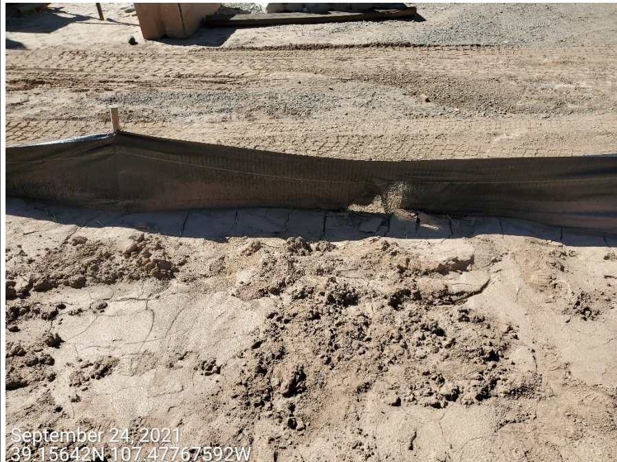
Photo 6: Photos taken from the western perimeter of the Location. Photo shows perimeter controls (silt fence) remain in improper functioning condition per good engineering practices.
