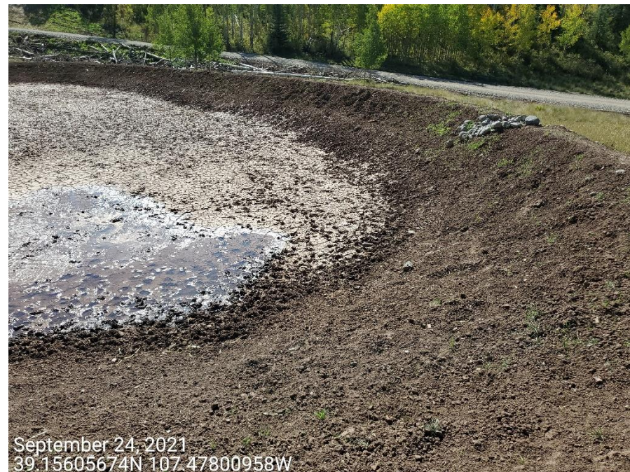
Photo 11: Photo provides overview of the sediment trap/pond to the west of the Location.
