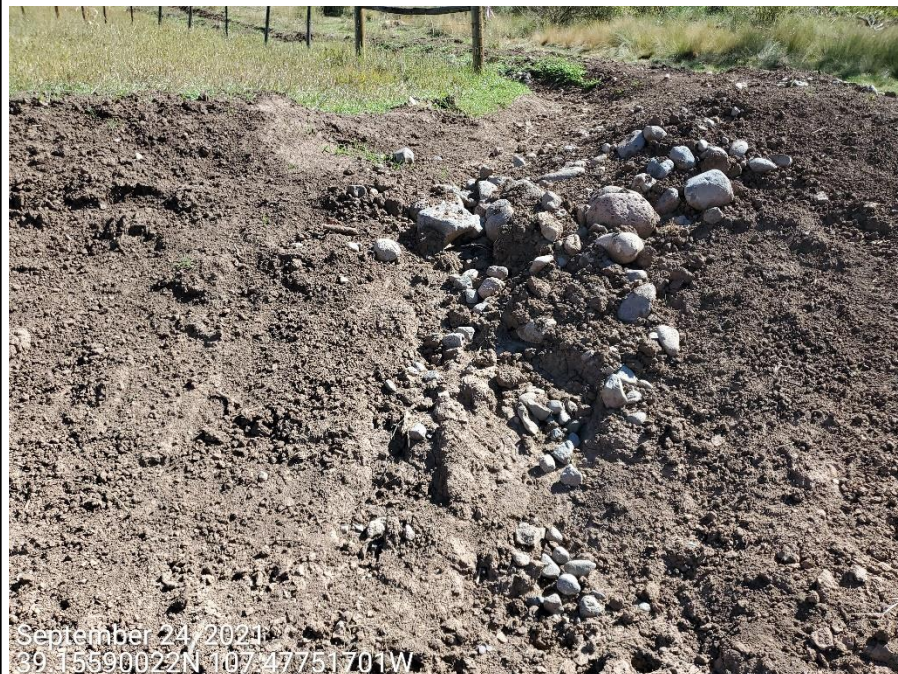
Photo 12: Photos taken from the sediment trap/pond west of the Location. Previous inspections documented that the inlets were inadequate. Photos show inlets remain inadequate per good engineering practices.
