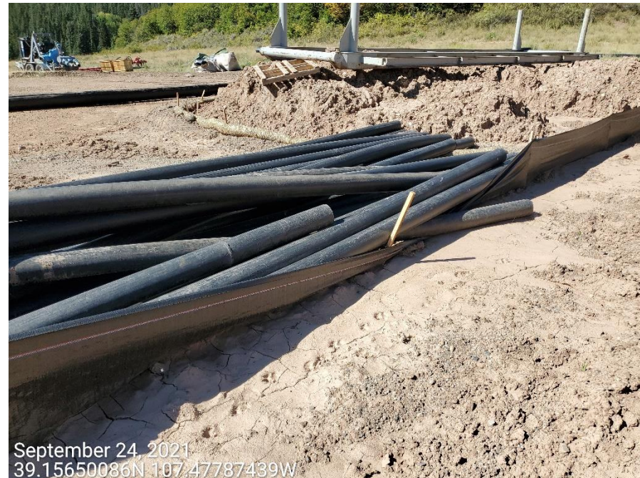
Photo 6: Photos taken from the western perimeter of the Location. Photo shows perimeter controls (silt fence) remain in improper functioning condition per good engineering practices.
