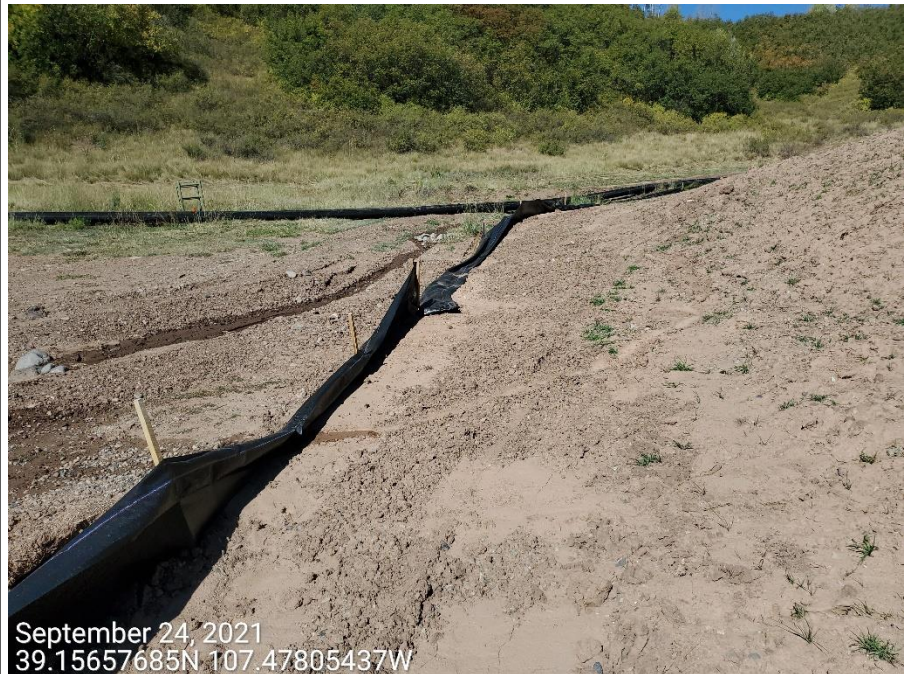
Photo 7: Photos taken from the western perimeter of the Location. Photo shows perimeter controls (silt fence) remain in improper functioning condition per good engineering practices.
