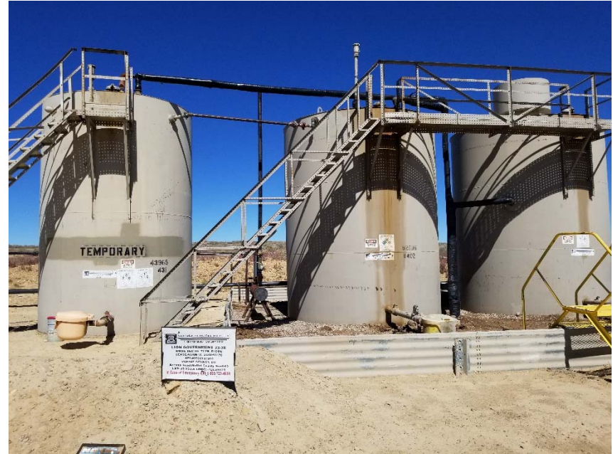
Photo 2. NFPA diamonds faded on tank labels.
