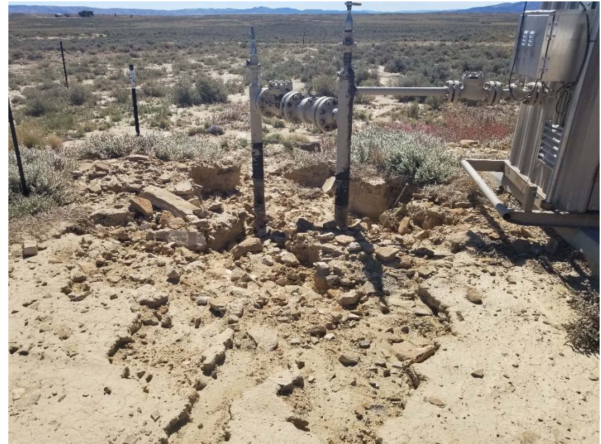
Photo 4. Erosion and sediment migration at location perimeter adjacent to gas meter run.
