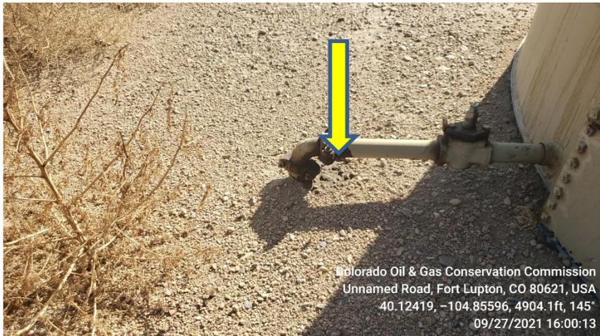
**Photo 17 Stained soil by Crude tank flow line**
