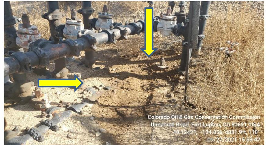
**Photo 10 Stained soil by the flow line manifold**
