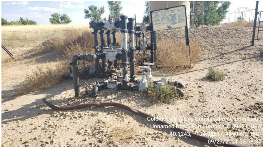
**Photo 9 Flow line manifold**
