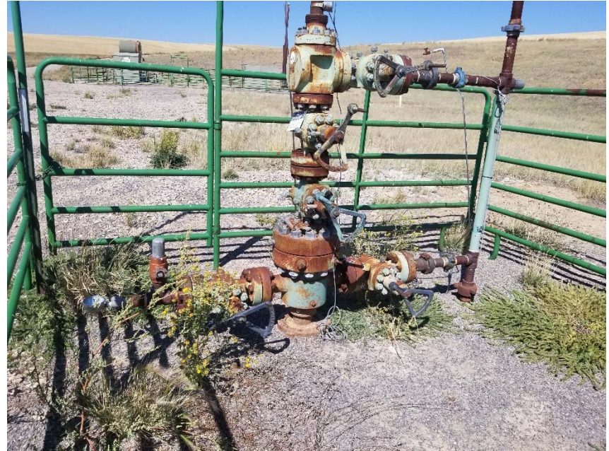
Photo 2. No bradenhead access apparent.
