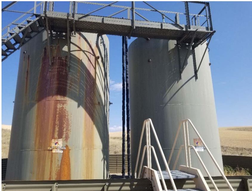
Photo 3. Holes in tank on left side labeled with 300 BBL capacity.
