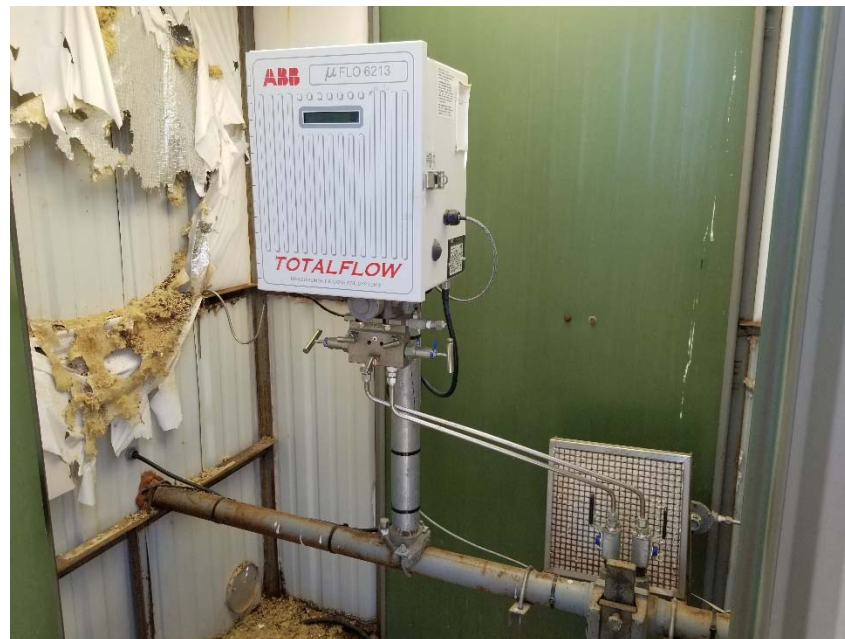
Photo 3. No calibration in gas meter run.
