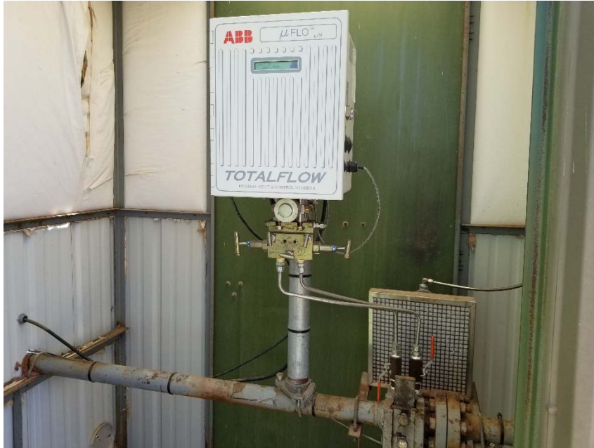
Photo 3. No calibration information in gas meter run.
