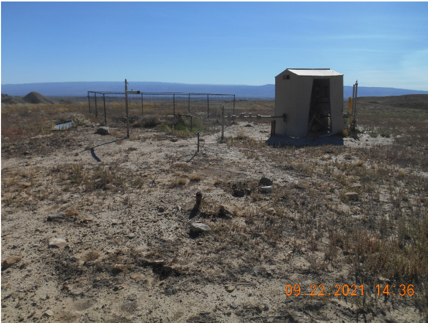
Meter housing and Pit on SW corner of location. Numerous flowline risers.
