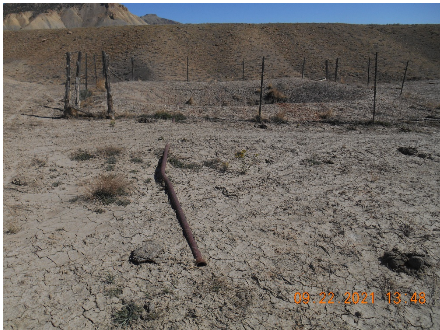
Pit on NE corner of location. Disconnected 2" flowline.
