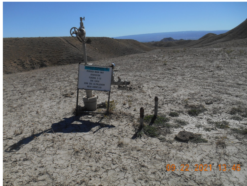
Wellhead with sign. 2-2" flowline risers
