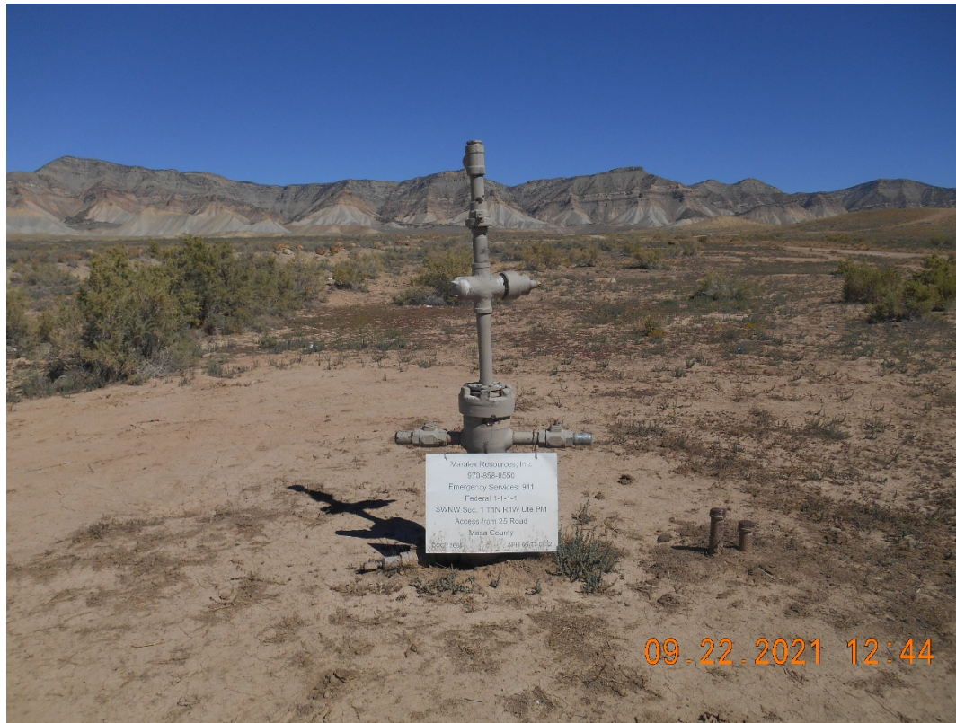
Wellhead with sign
