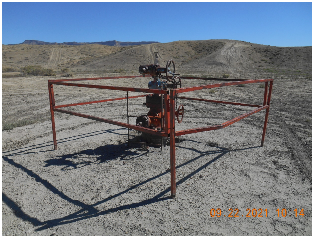
SI/TA wellhead with fence. Missing sign.
