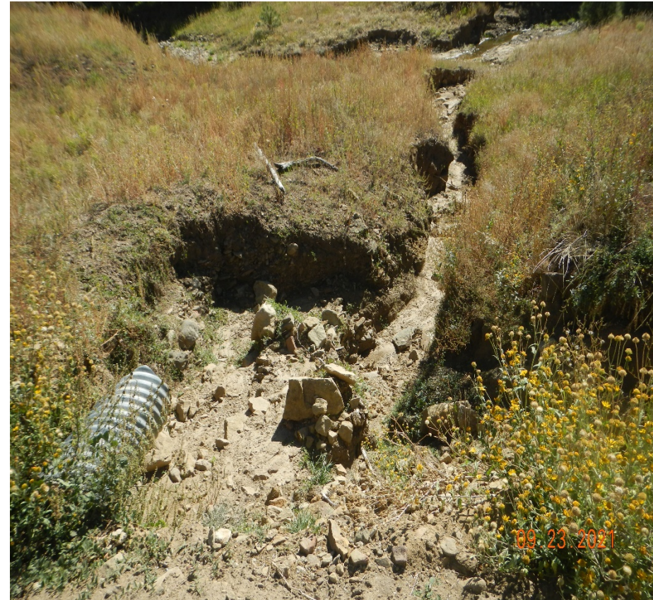
Photo 4. The culvert outlet is eroded and does not have outlet protection.
