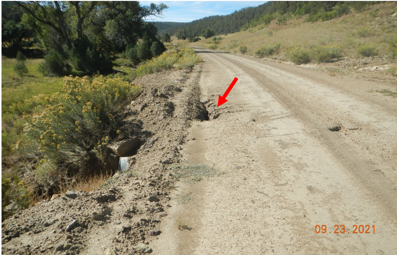
Photo 1. Facing southwest along the main road in the canyon. The road has been graded however, there is still culvert maintenance needed. Red arrow points to erosion undercutting by the culvert which will end up eroding.
