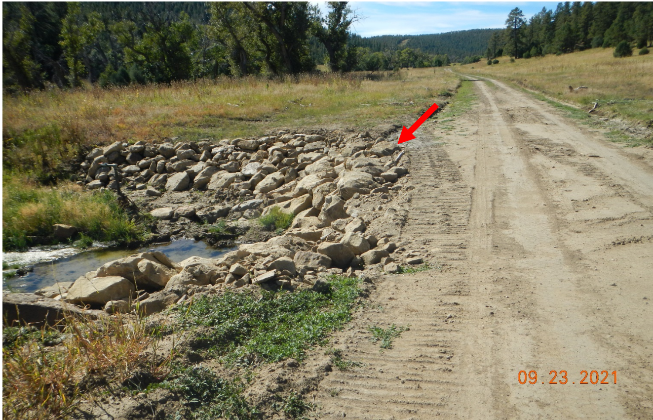
Photo 2. This culvert outlet has been repaired with rock armoring. One issue is observed, there is no diversion for stormwater off the road shown at red arrow which will cause stormwater to pool in this area.
