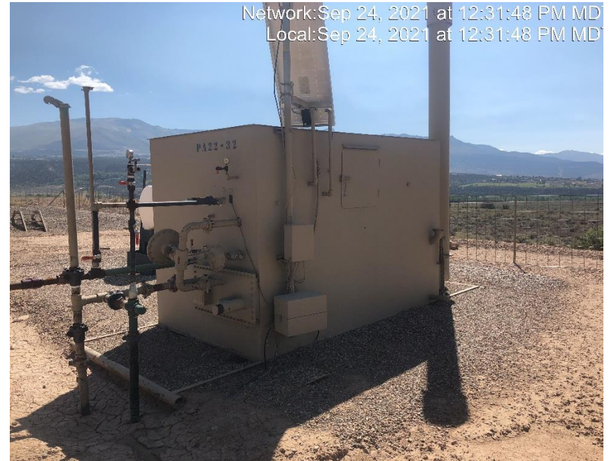
Photo #4950 Glycol storage tank missing required information.
