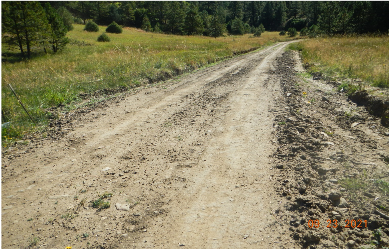
Photo 2. The culvert along the road are filled in with sediment causing stormwater to flow down the side of the road. Lat/Long:37.00499,-104.83742. Previous corrective action was not completed.
