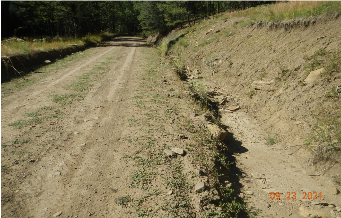
Photo 4. Further up the road in the canyon is erosion along the roadside with insufficient BMP's.
