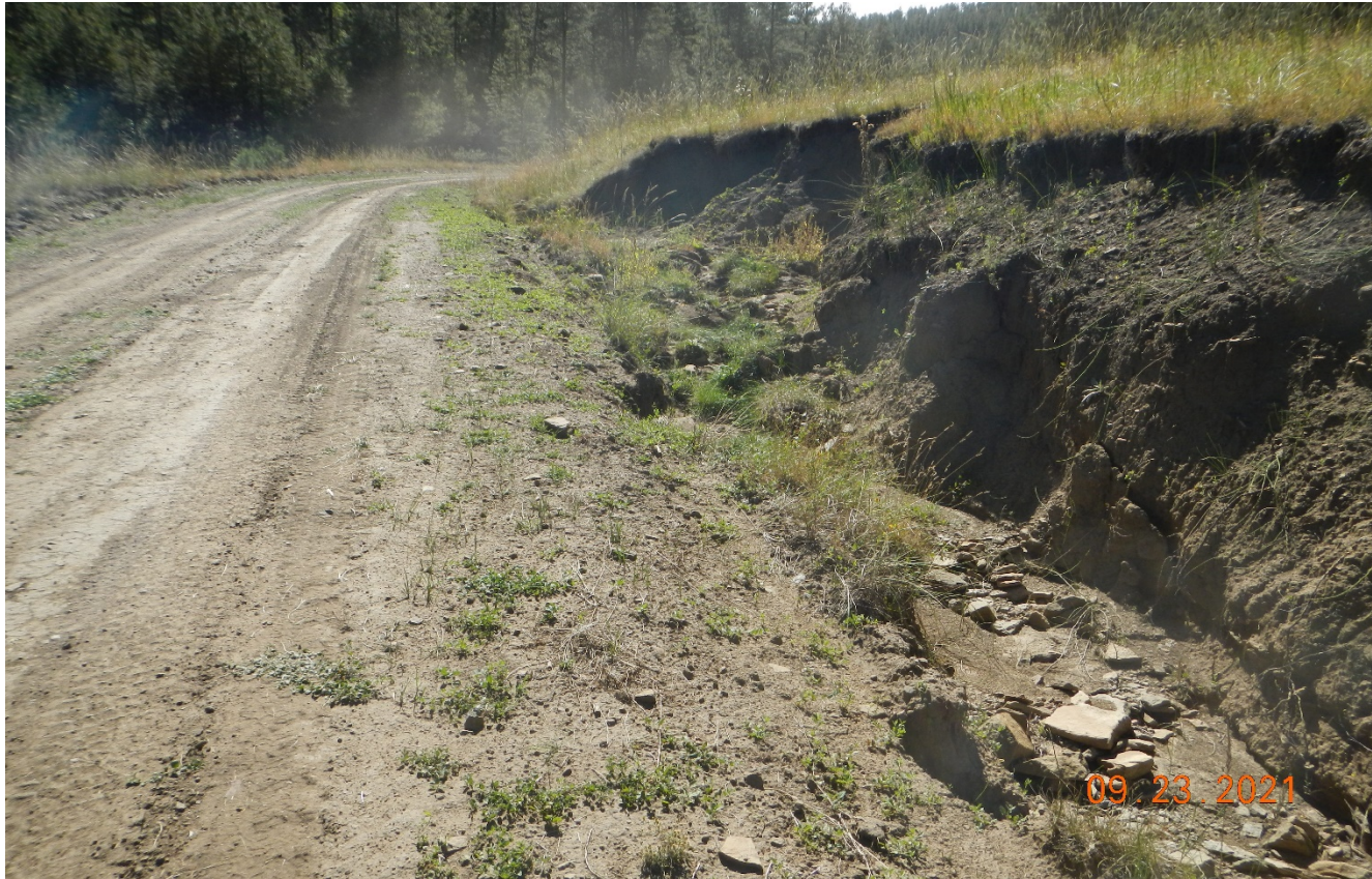
Photo 3. The side of the road is eroded and not stabilized at Lat/Long:36.99952,-104.83425. This area needs to be resloped, seeded, and stabilized.
