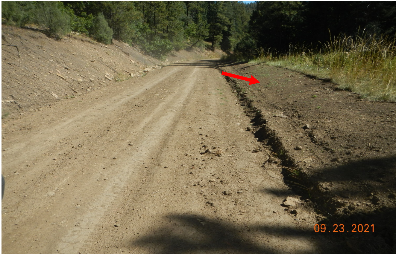
Photo 5. There was grading performed along the road. The disturbance along the side of the road shown at red arrow needs to be seeded and reclaimed.
