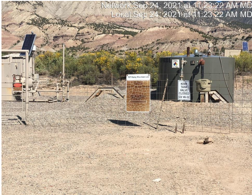
Photo #4948 Battery sign weathered and not legible.
