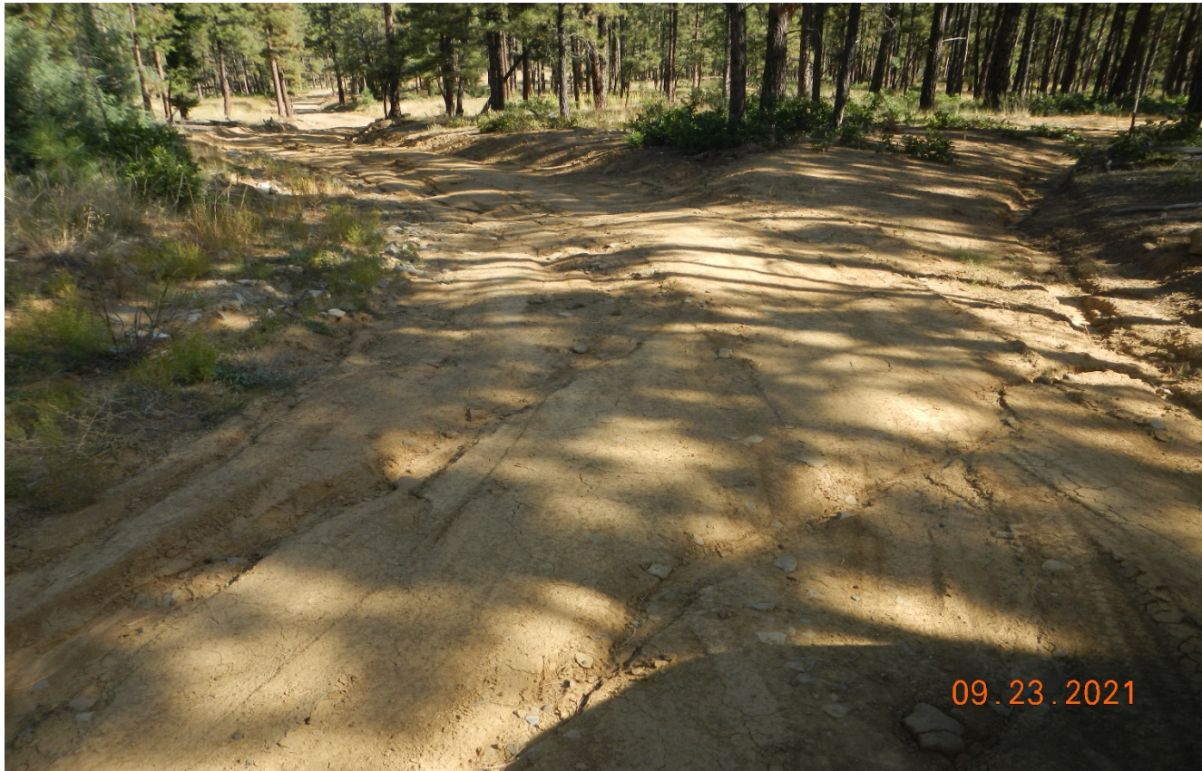
Photo 1. Facing north toward the access road. There is a berm and runoff ditch in this area of the road. There is sign stormwater is still directed down the road causing erosion.
