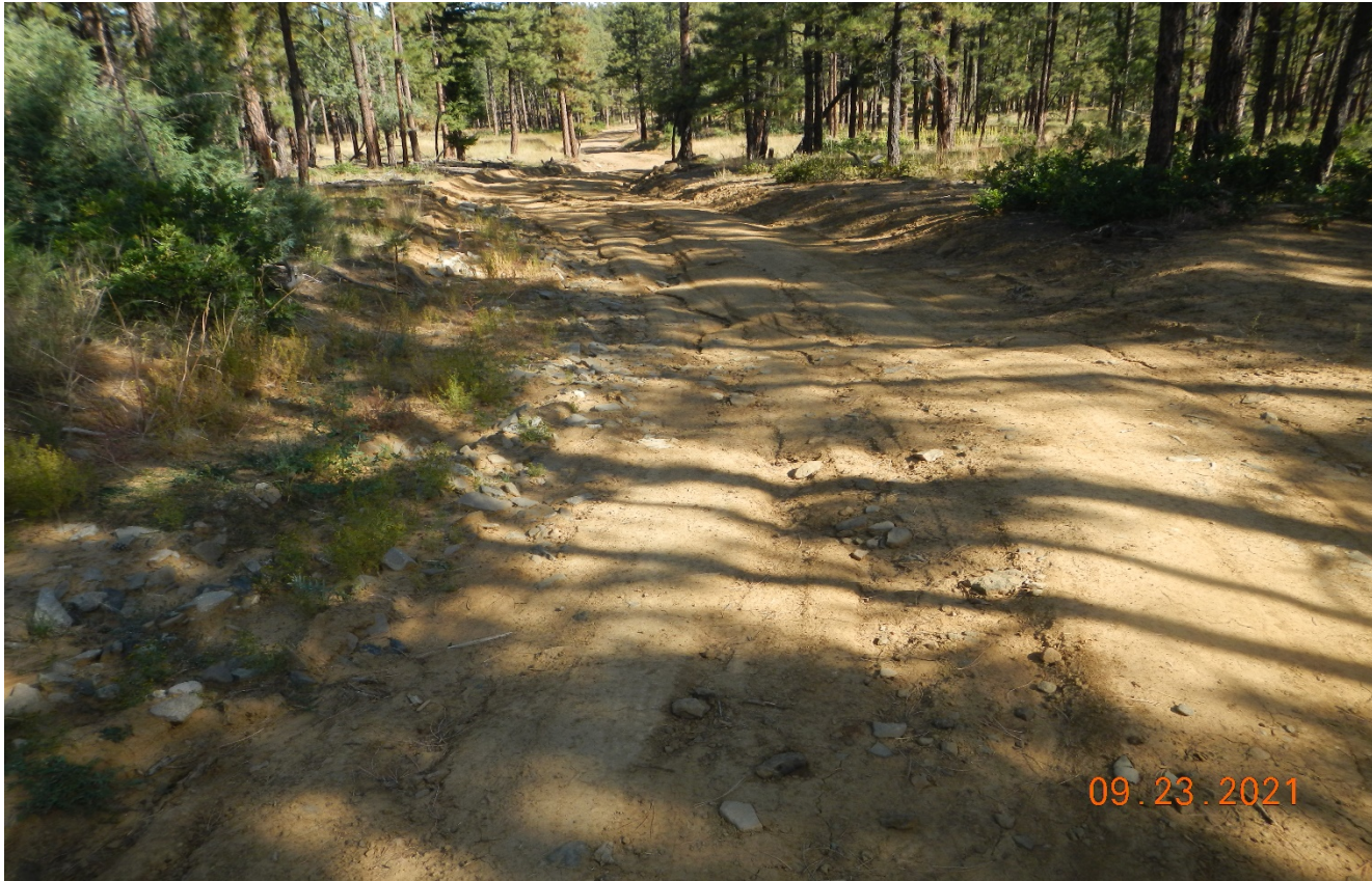
Photo 2. Stormwater directed down the road has caused erosion and degradation of the road.
