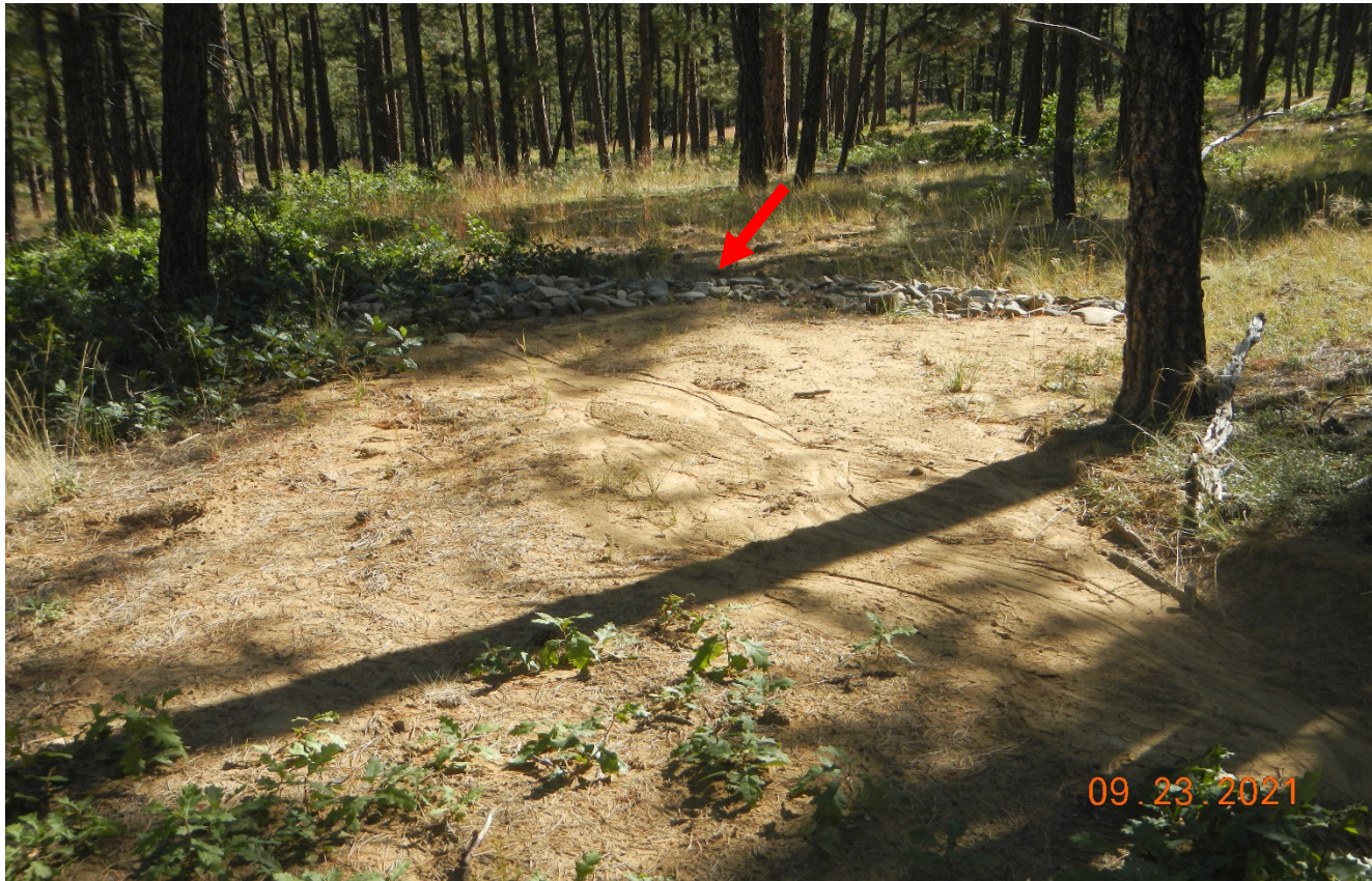
Photo 3. A rock rip/rap structure was installed since previous inspection which has contained sediment from the road. This sediment will need to be cleaned out. A sediment trap would be more appropriate in this area.
