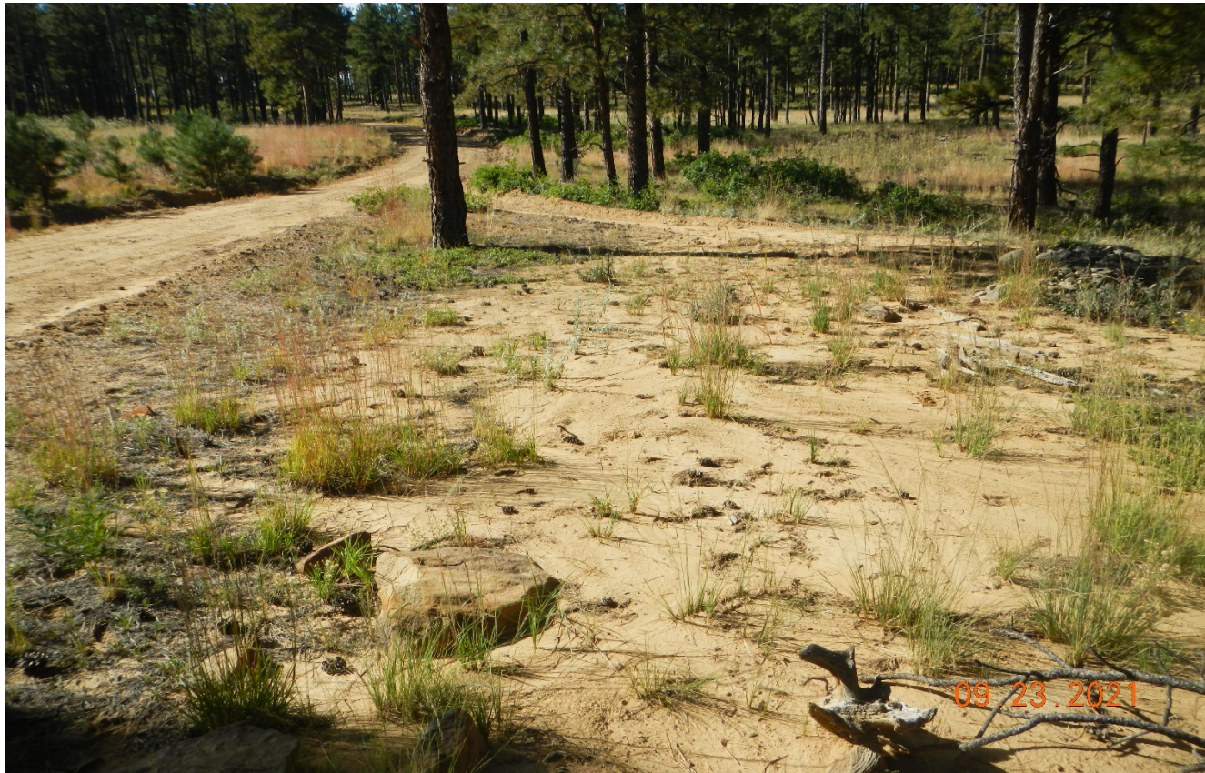
Photo 4. Facing south adjacent to the access road. This photo shows the sediment deposition off the road into the adjacent area. The road needs to be stabilized to prevent erosion.
