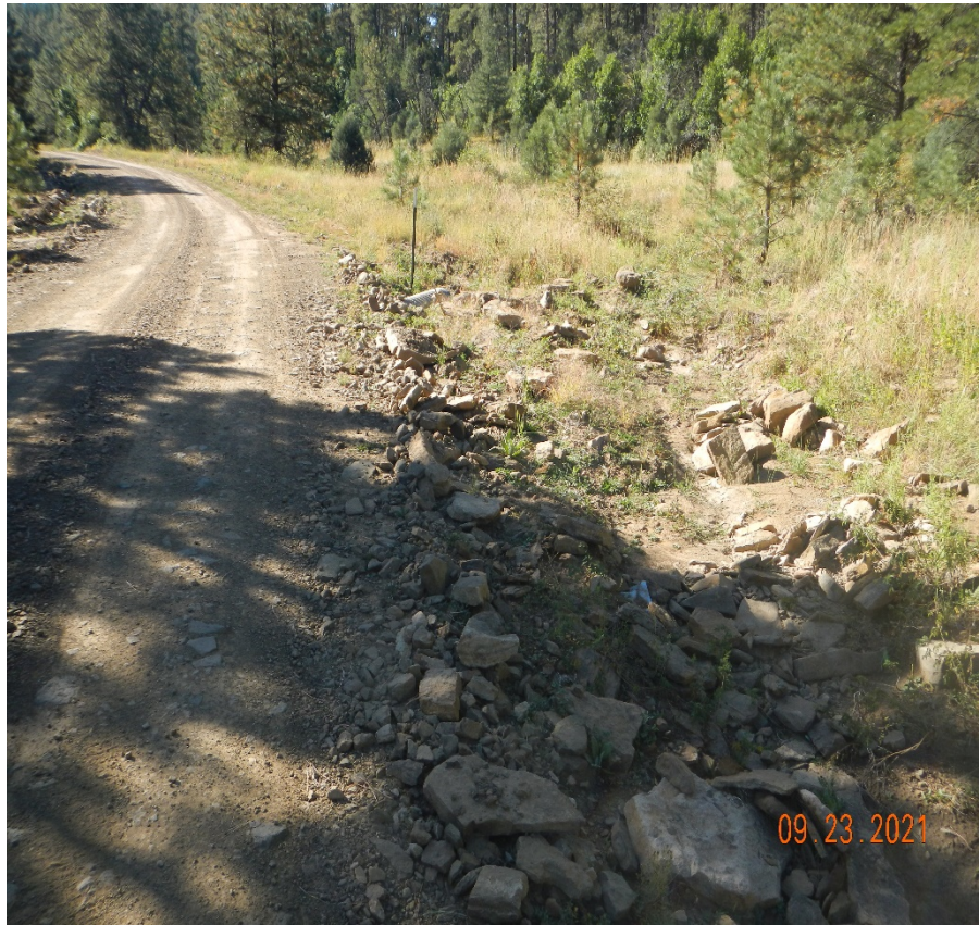
Photo 1. Facing southeast along the main road in the canyon. This culvert is filled in with sediment causing stormwater to flow down the side of the road.
