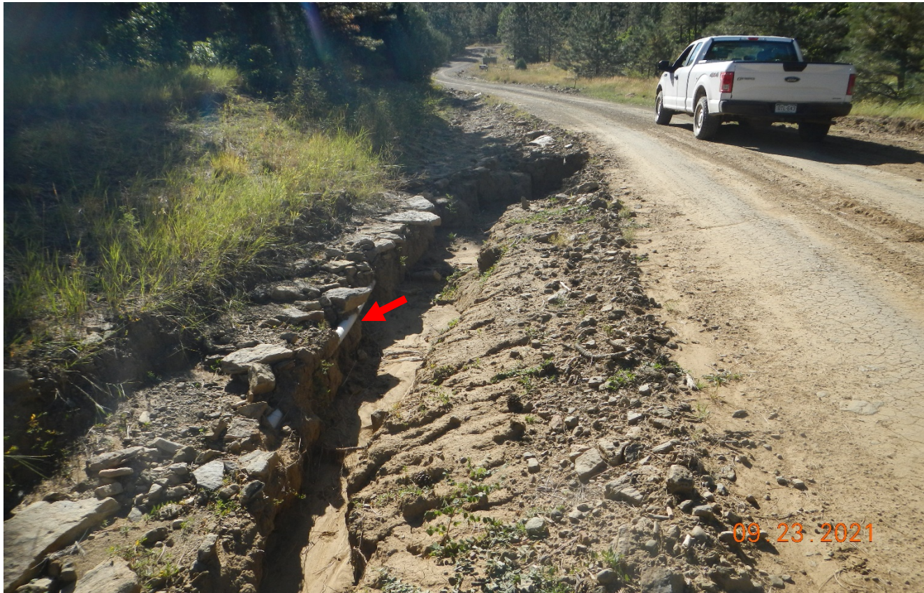
Photo 4. Further along the road is areas of erosion. There is an exposed pipeline which needs to be covered and protected.
