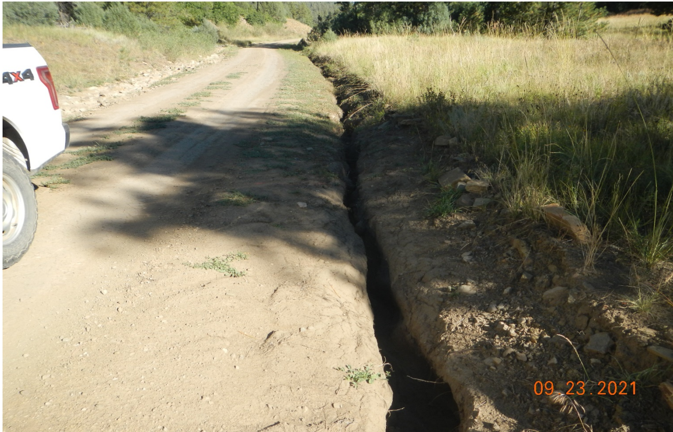
Photo 3. Stormwater is causing a deep erosion channel along the side of the road which needs to be repaired.
