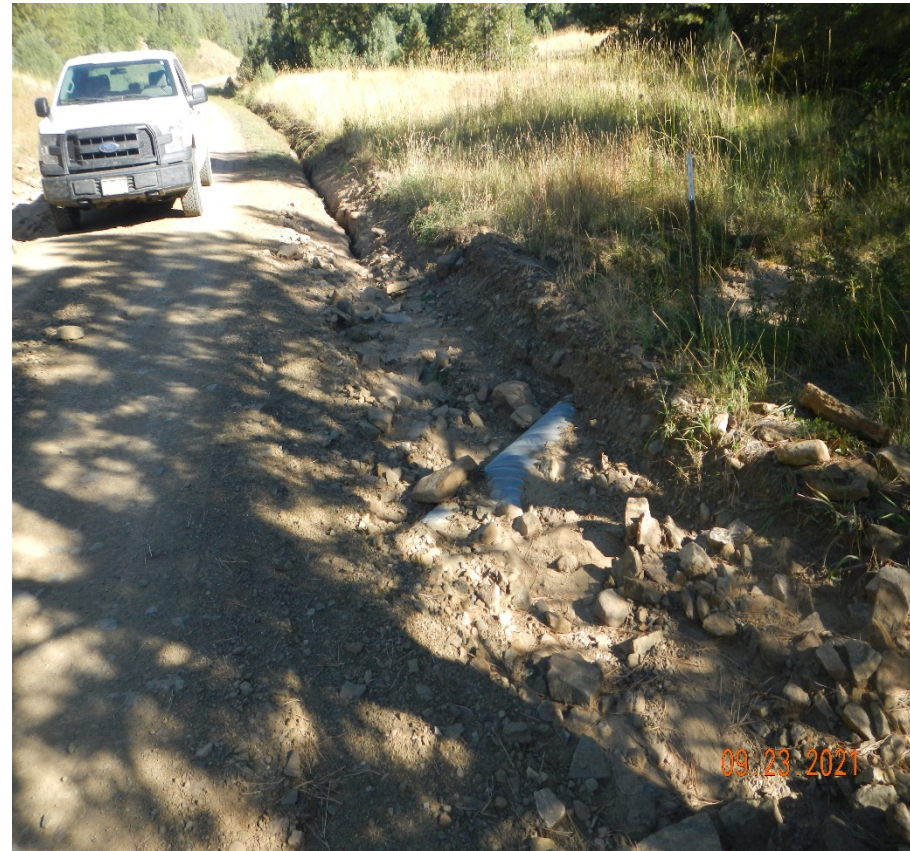
Photo 2. Facing northwest at the same culvert outlet which shows stormwater is flowing past the culvert causing erosion of the road.
