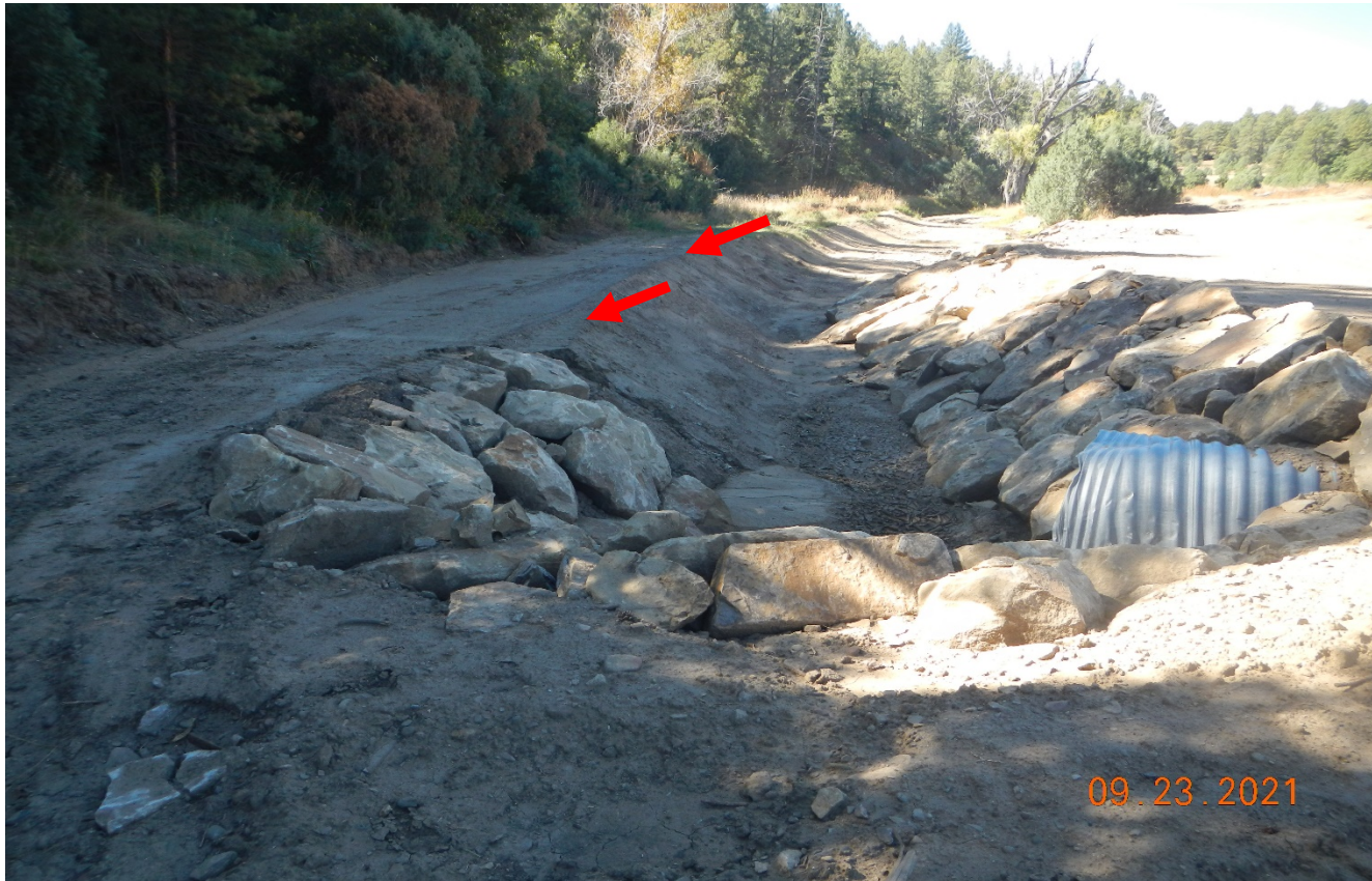
Photo 4. Facing at south side of the road at the additional culvert inlet. Disturbed bare shown at red arrow will need to be seeded and stabilized.
