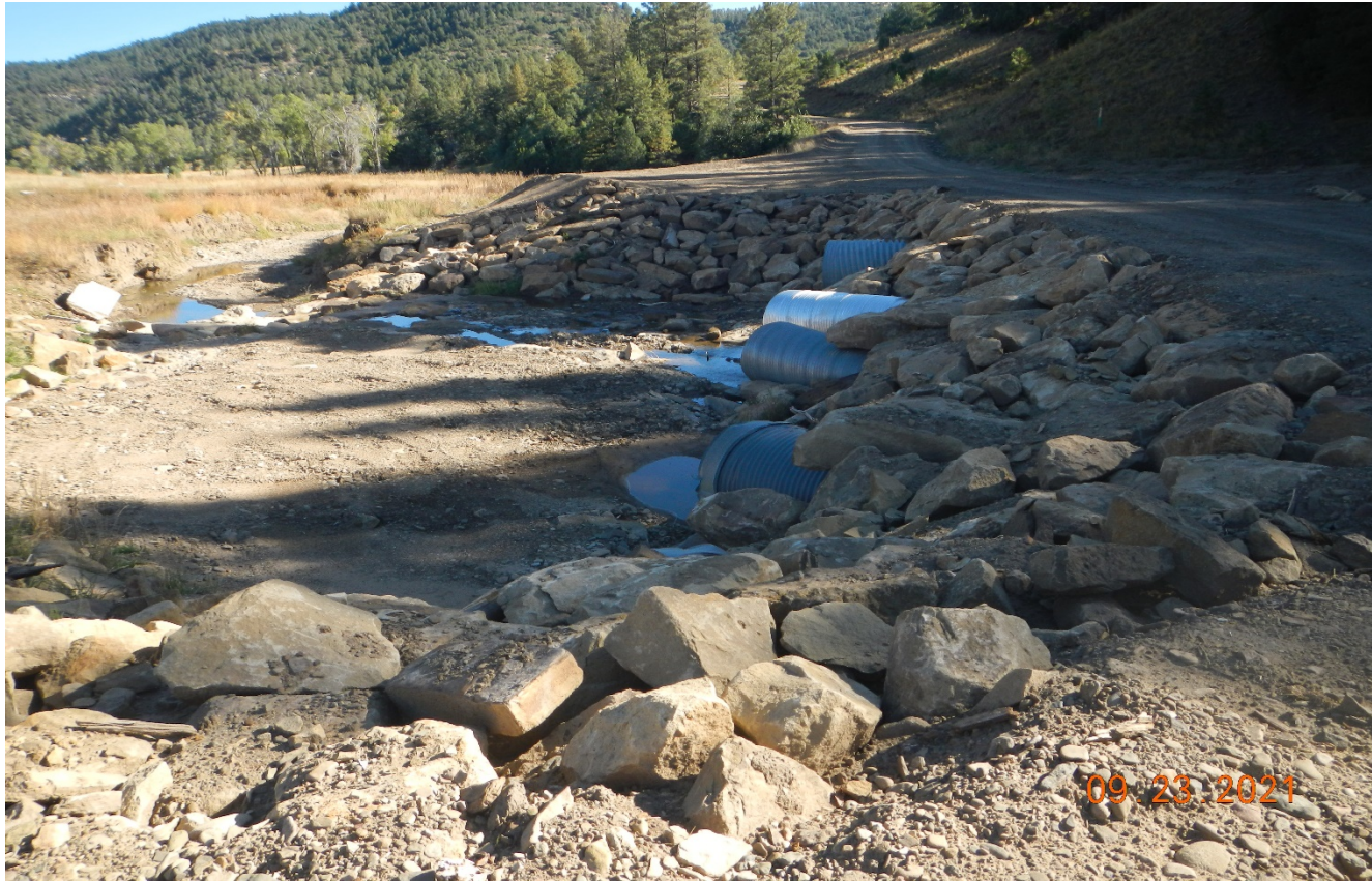
Photo 3. Facing toward the culvert outlets which are armored with rock rip/rap.
