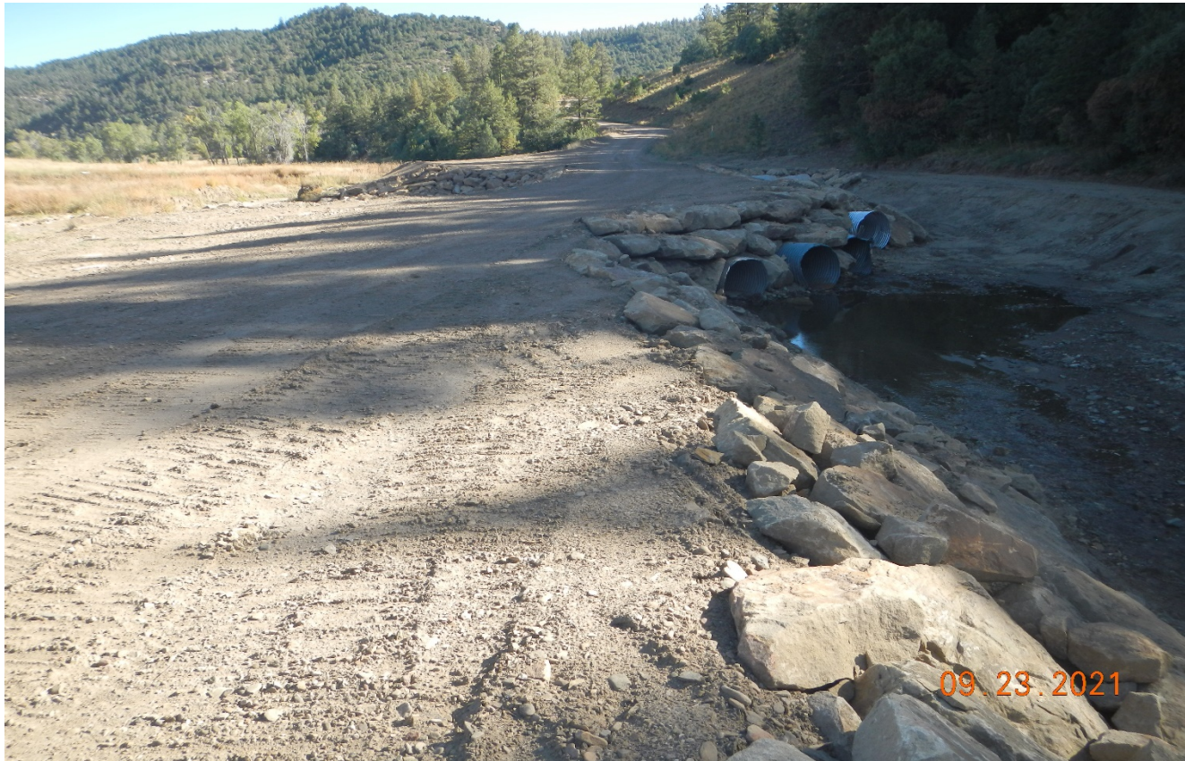
Photo 1. Facing northeast at the Lorencito creek crossing. The crossing has been repaired with an additional culvert installed.
