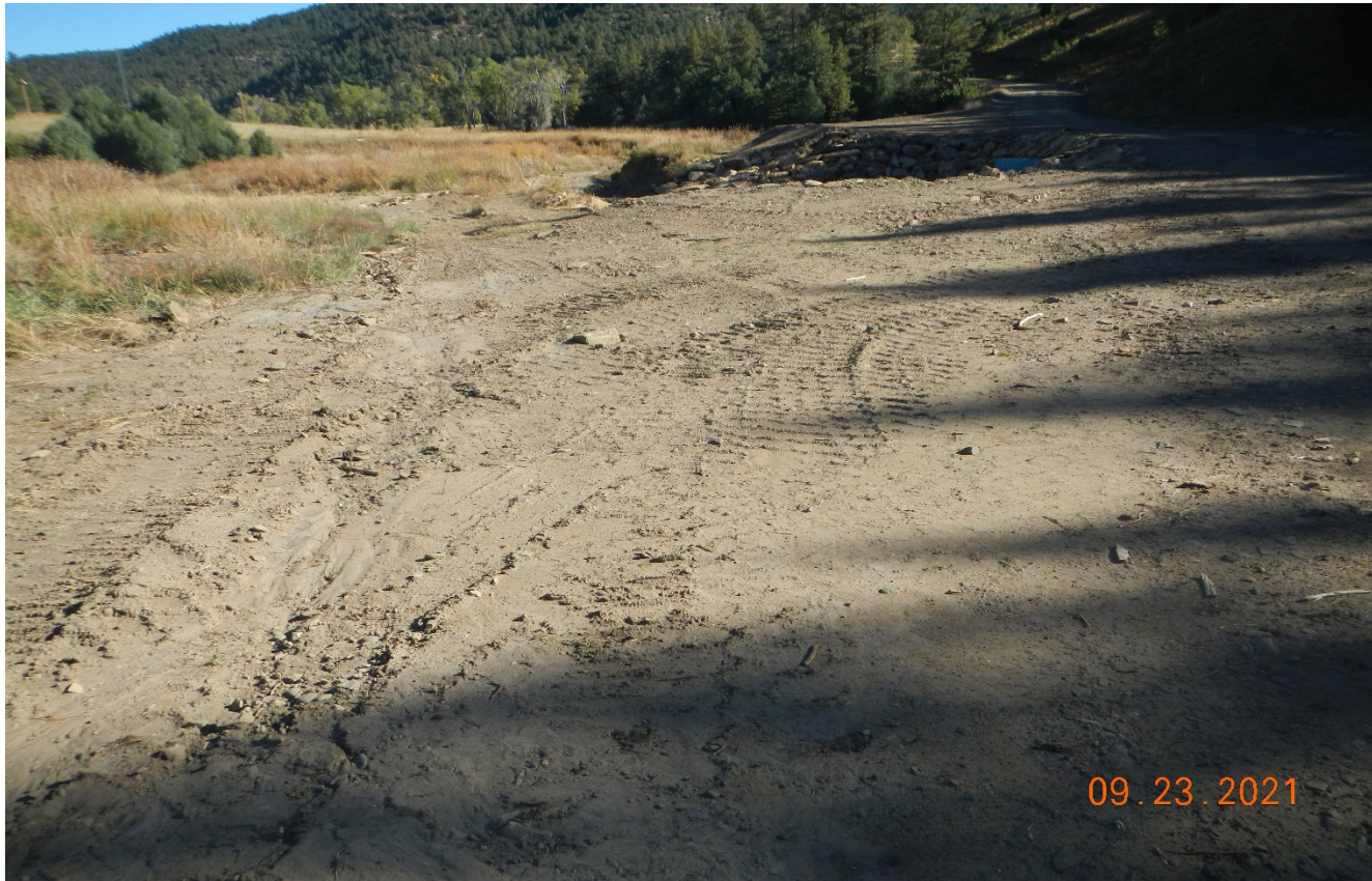
Photo 2. The disturbed bare soils along the roadside will need to be seeded and stabilized.
