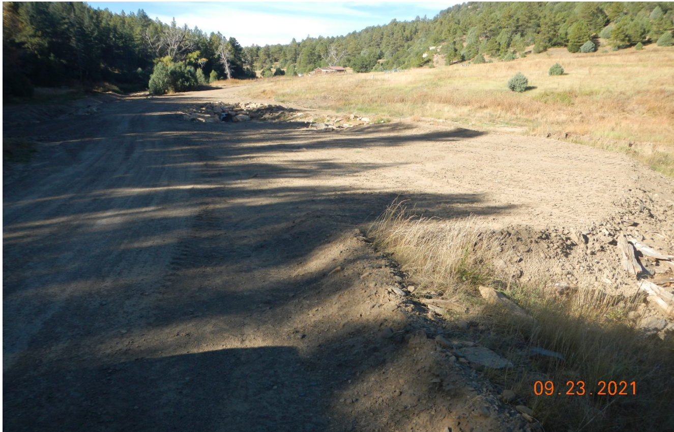
Photo 5. Facing back west at the Lorencito stream crossing which was repaired. The disturbed bare soils along the roadside will need to be seeded and stabilized.
