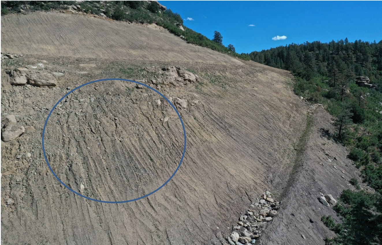
Photo 5. There appears to be signs of erosion in the area circled. This area may need additional BMP's to prevent erosion.
