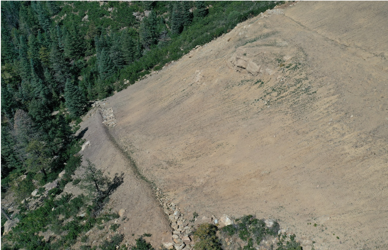
Photo 3. Facing west down at the location. A large berm was installed at the bottom of the location.
