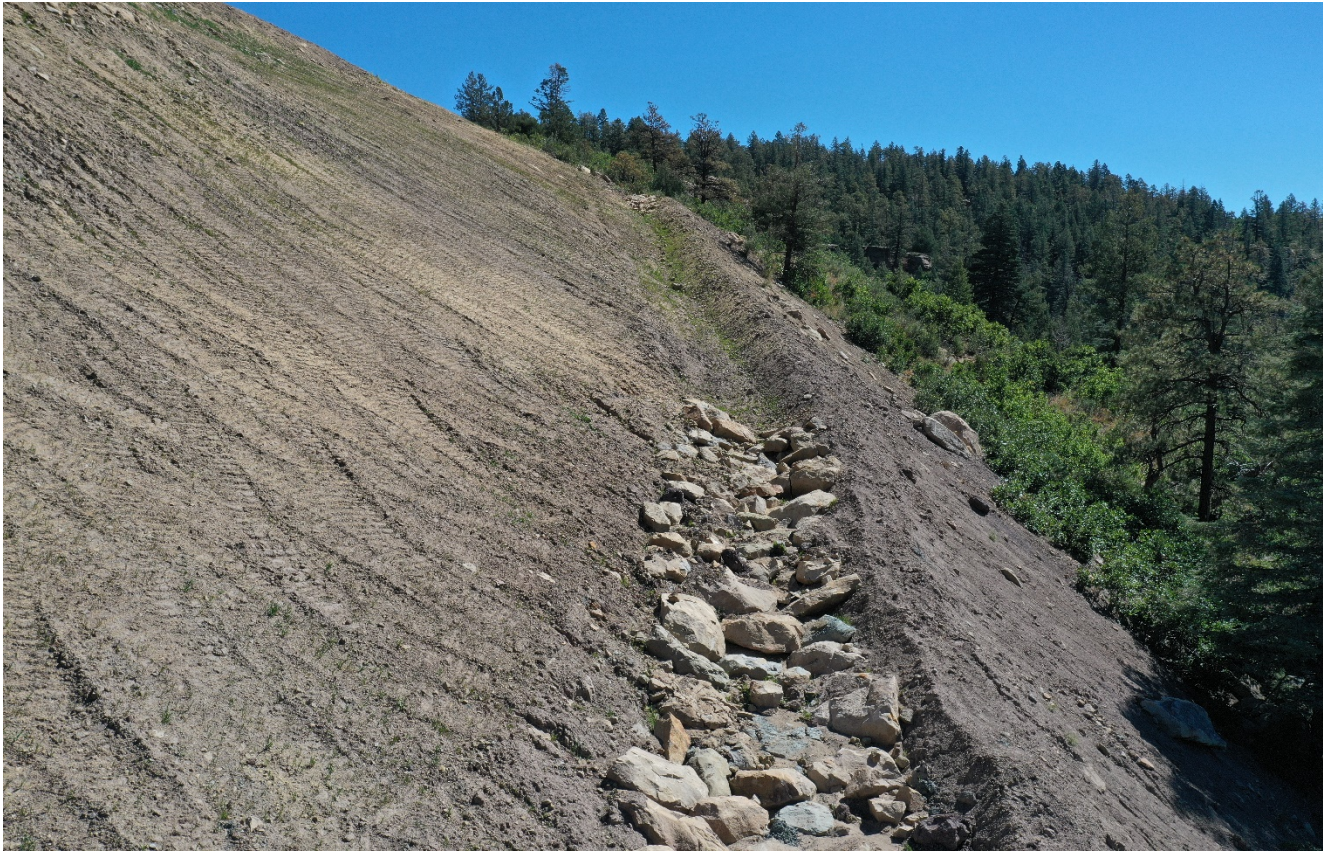
Photo 6. Facing east at the bottom of the location. A large berm was installed at the bottom with rock rip/rap.
