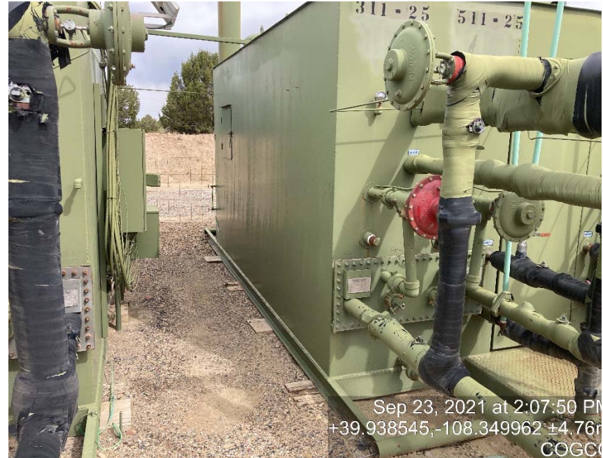
Lack of labeling on glycol vessel
