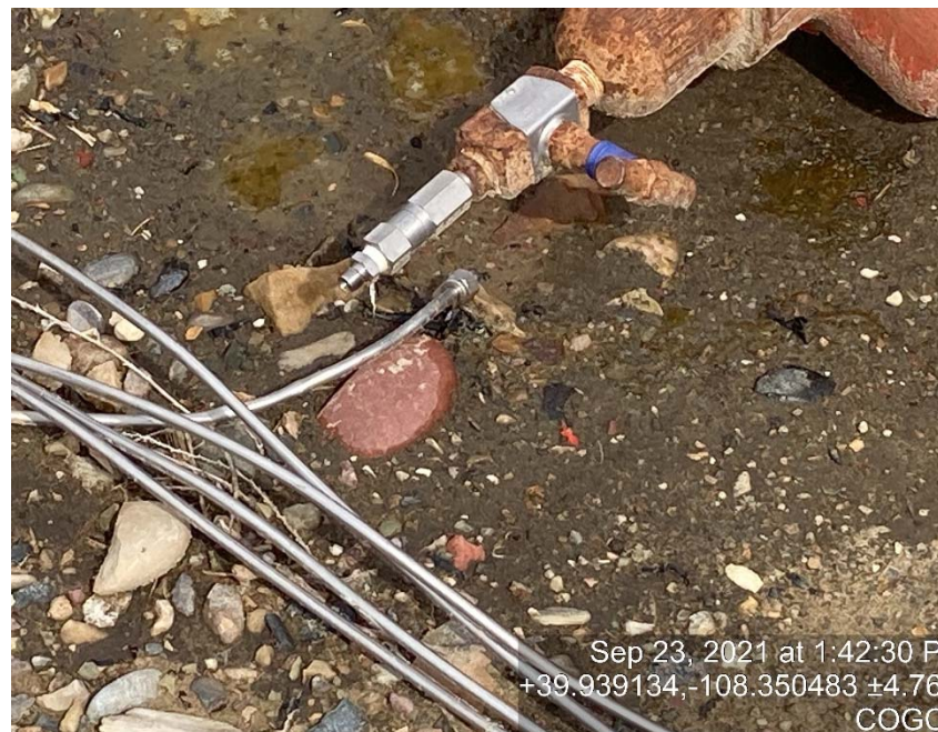
Staining and chemical line disconnected
