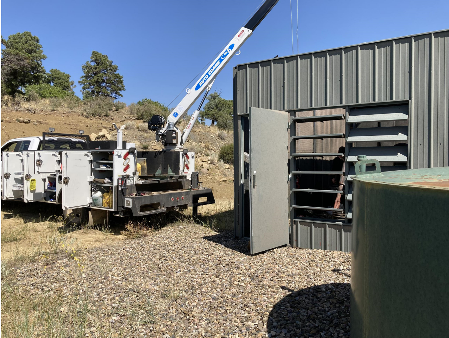
PHOTO 1: THE COMPRESSOR ENGINE WAS SCHEDULED FOR AN ENGINE SWAP ON 09/17/21, WHICH WAS COMPLETED.
