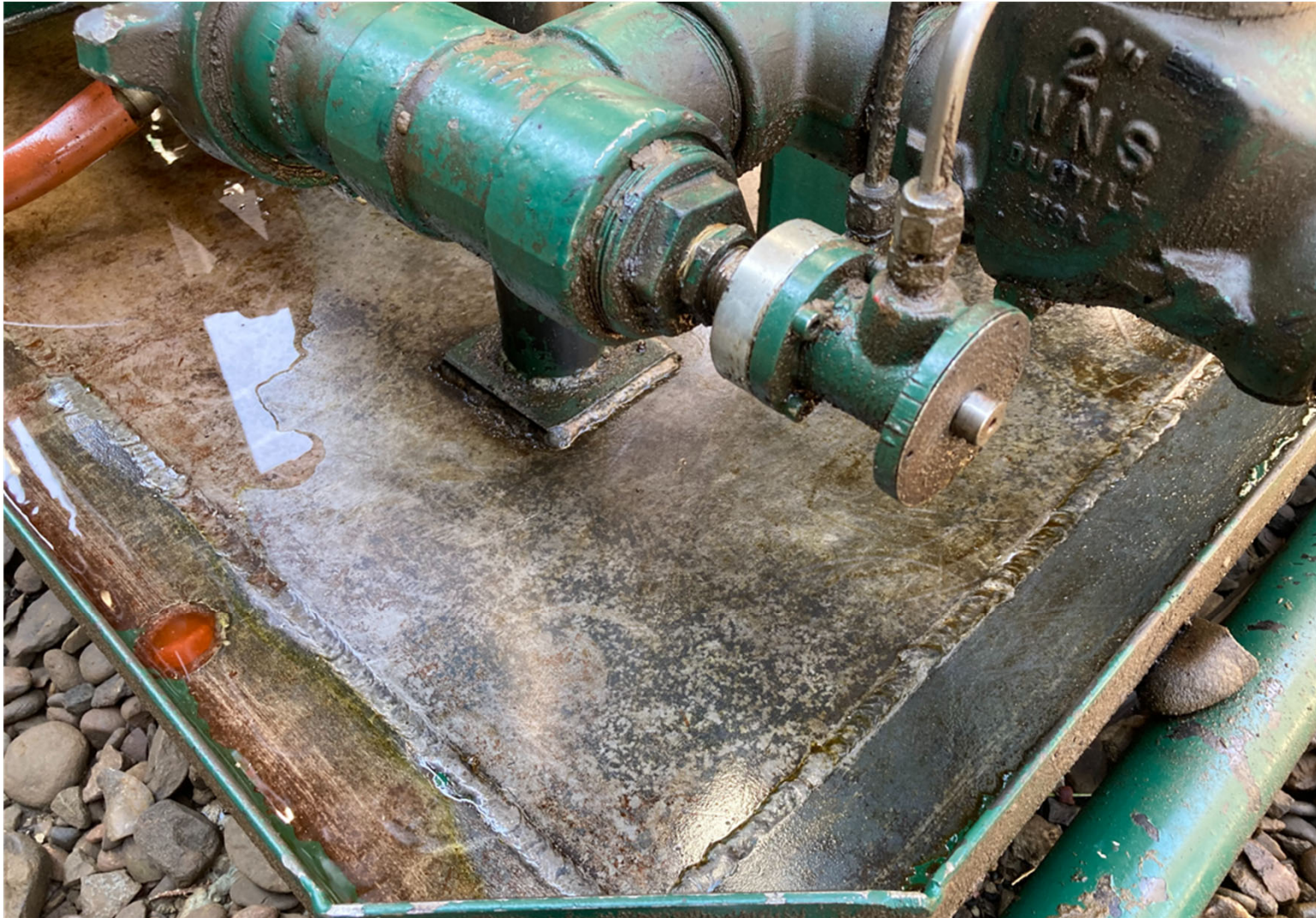
PHOTO 2: THE FLUID IN THE CONTAINMENT OF THE LIQUID RING PRIMARILY CONSISTED OF RAIN WATER FROM THE STORM ON TUESDAY NIGHT 9/14/21. THIS FLUID WAS REMOVED ON 09/16/21.
