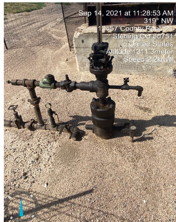
2. Wellhead with casing disconnected from flowline.
