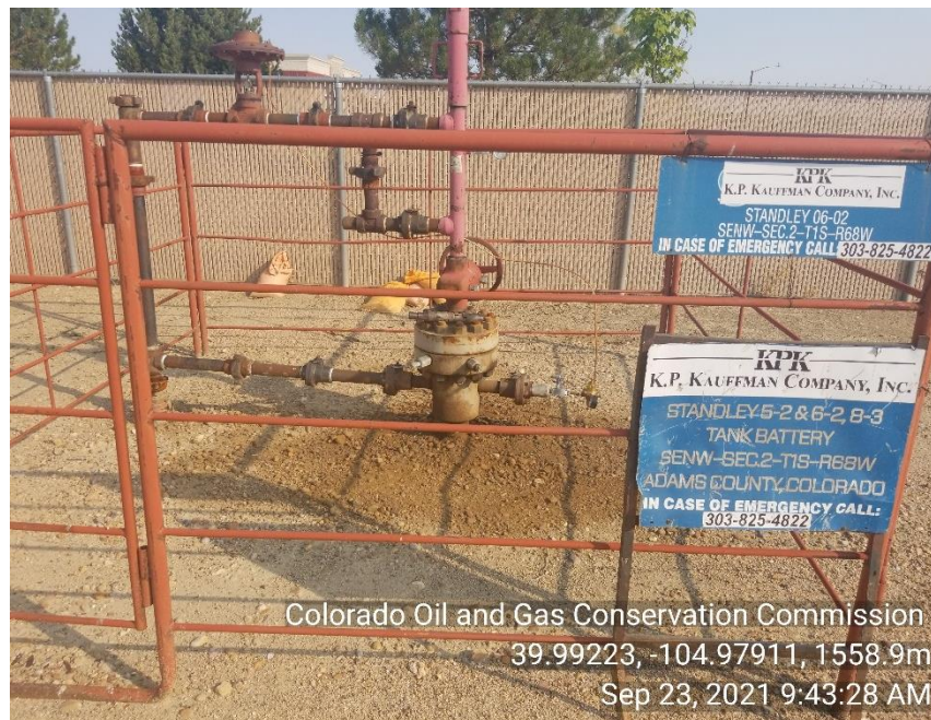
Photo 5 Stained soil around 6-2 well head Flow lines from well head appear to be in the closed position.
