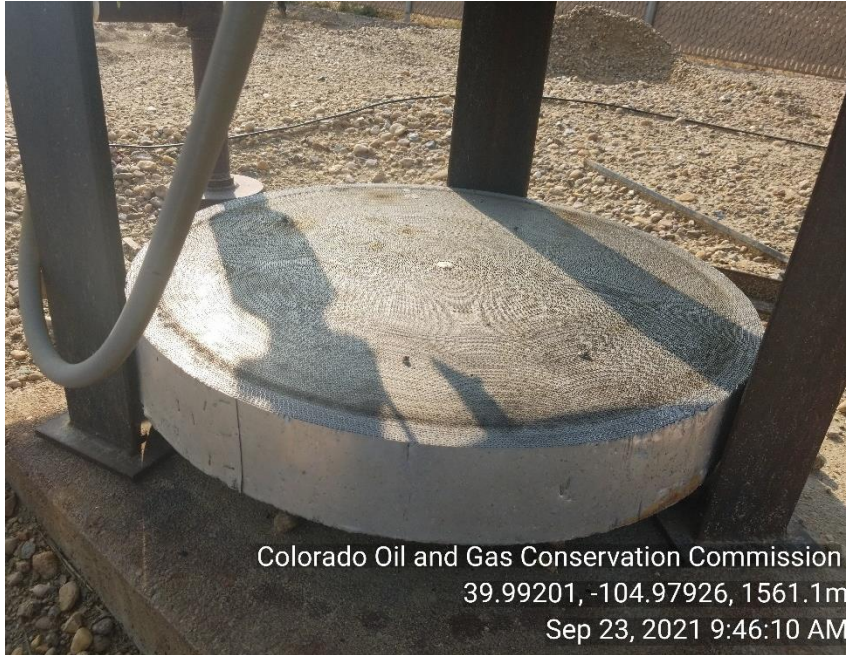
Photo 9 ECD fire arrester on ground
