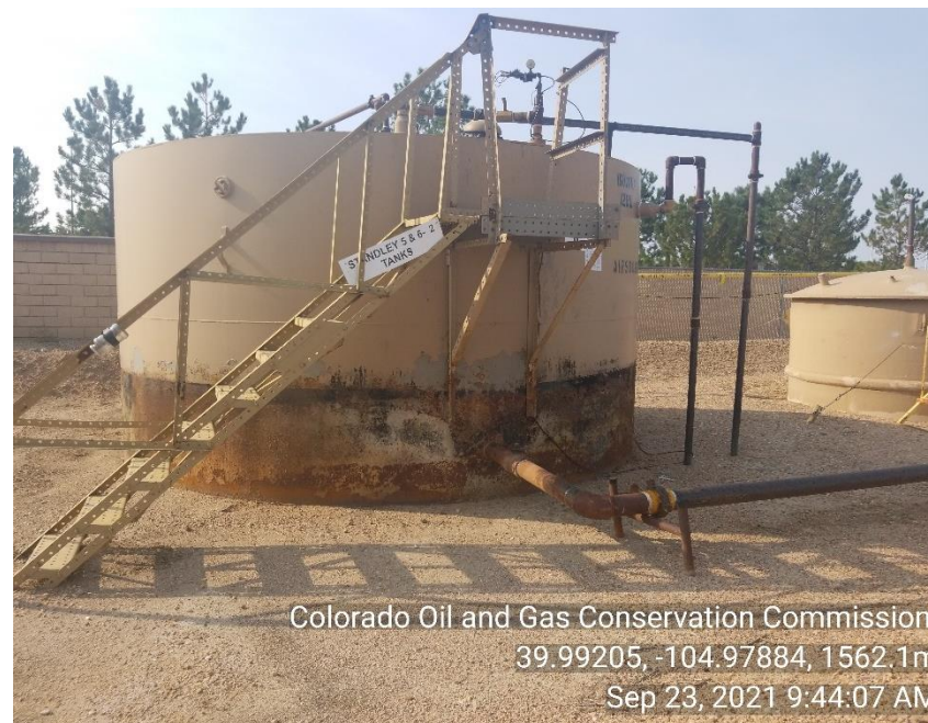
Photo 6 Crude oil tank next to public road and bottom half of tank appears to be rusting.
