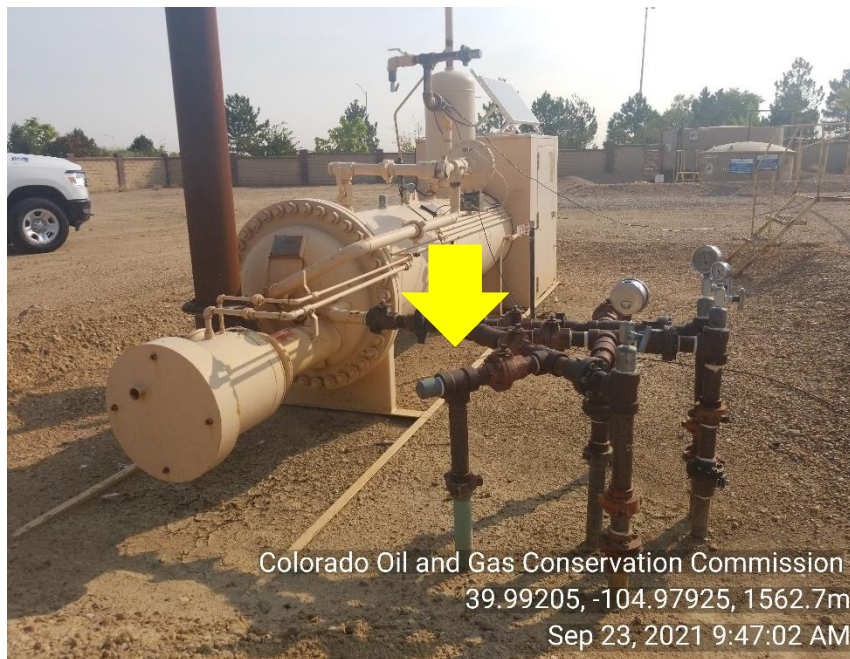
Photo 11 Sales line from separator has 2" bull plug installed
