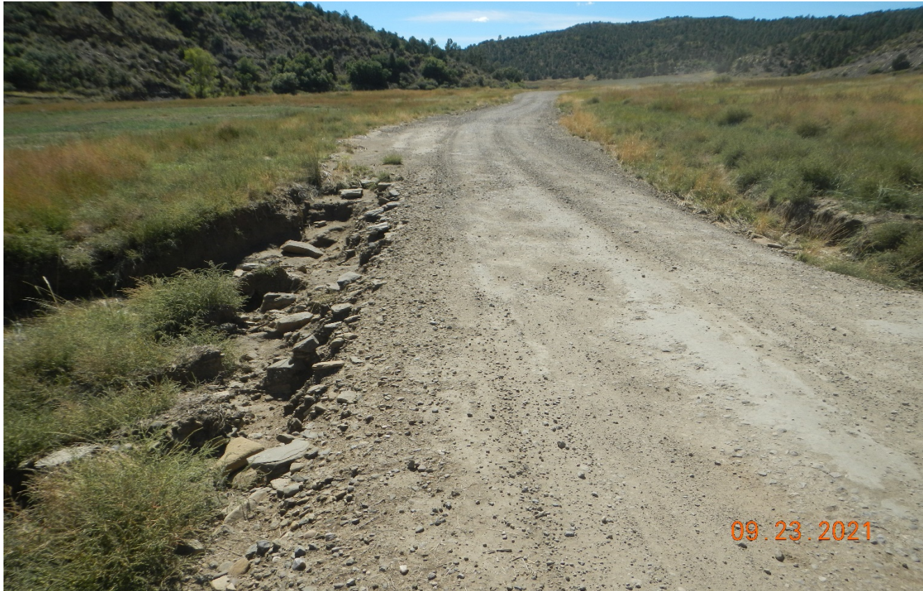
Photo 3. Further along the main road. Stormwater has caused erosion along the roadside. This area may need a culvert.
