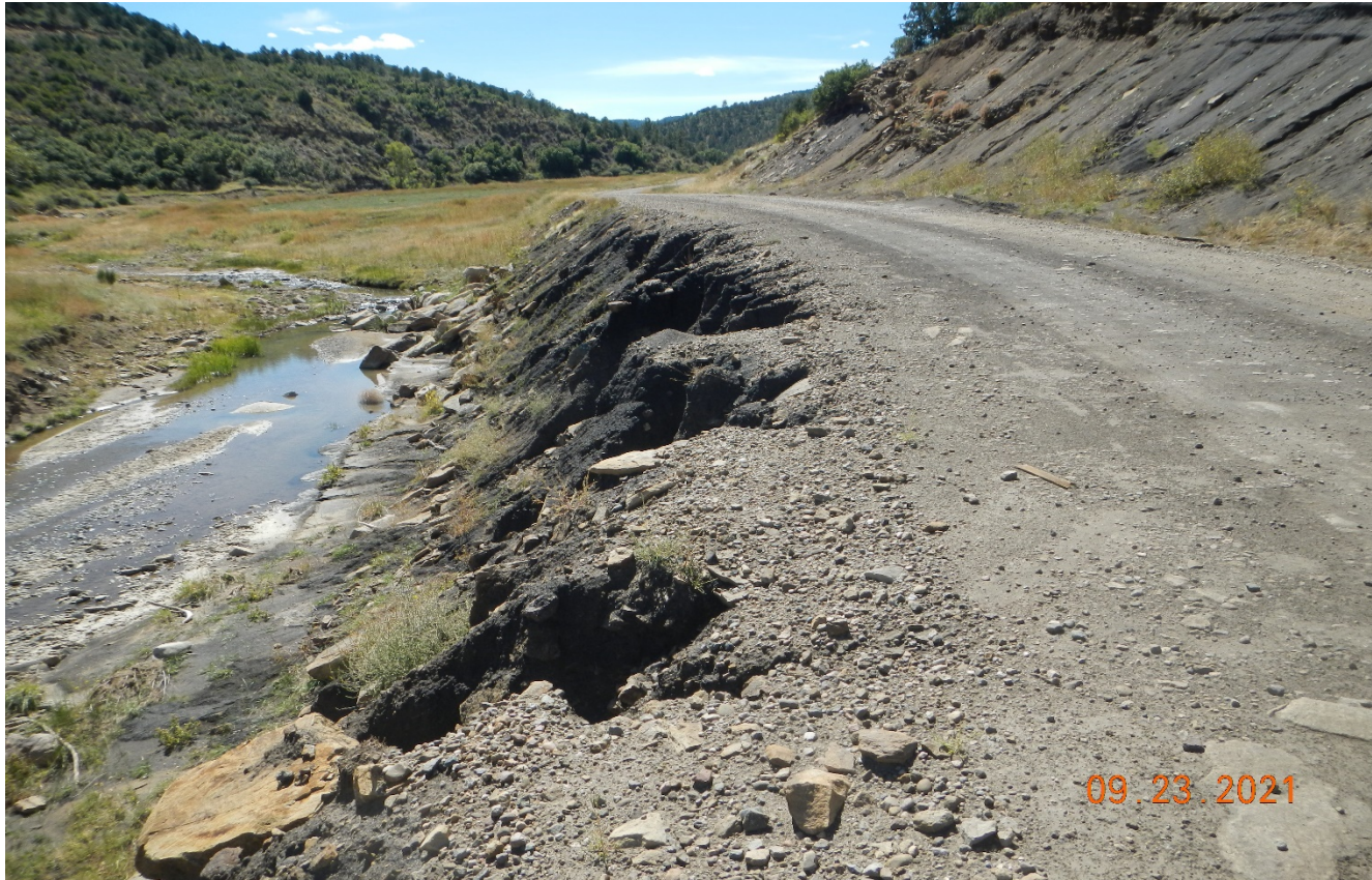
Photo 2. The side of the main road is eroded and not stabilized. Lat/Long:37.10084,-104.789327.
