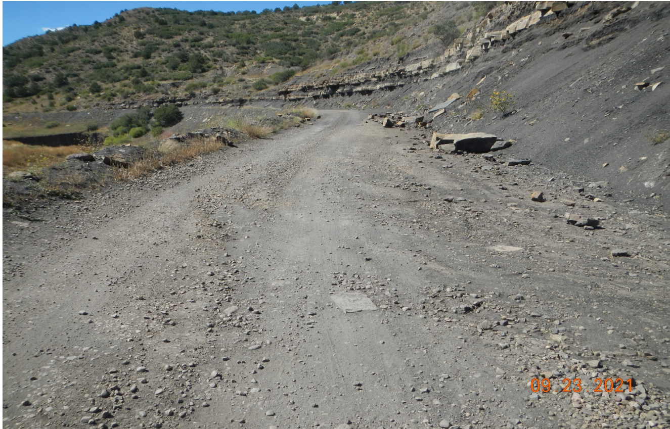
Photo 1. Facing southwest along the main road. There is rocks that have fallen into the road way.
