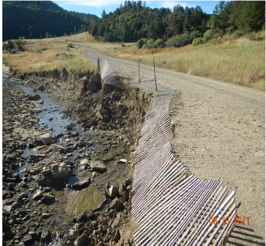
Photo 4. The side of the main road has eroded and is unstable. This area needs to be repaired and stabilized.
