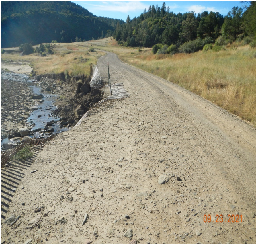
Photo 4. The side of the main road has eroded and is unstable. This area needs to be repaired and stabilized.
