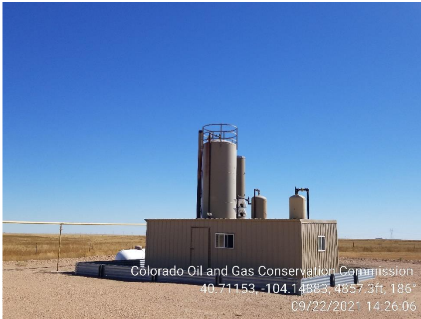
Photo 5 – South Heater Treater
