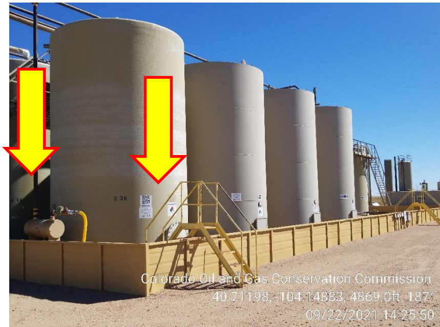
Photo 3 – North H2O Tanks missing Labels
