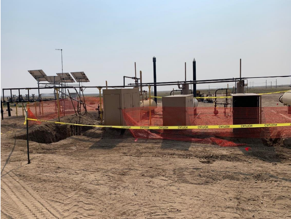
Impacted soil being removed and dumphine exposed
