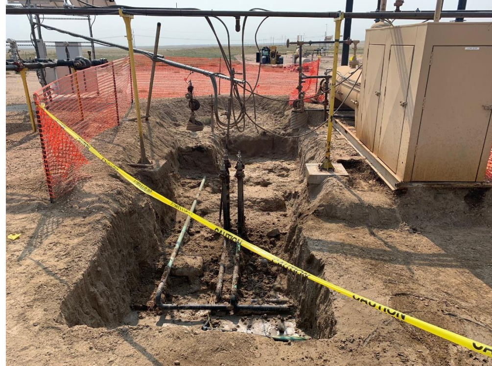
Impacted soil being removed and dumphine exposed
