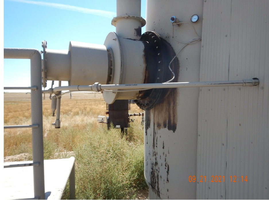
Photo 5. Photo taken from the southern tank battery, facing South. Photo illustrates equipment is not in good mechanical condition and is leaking.
